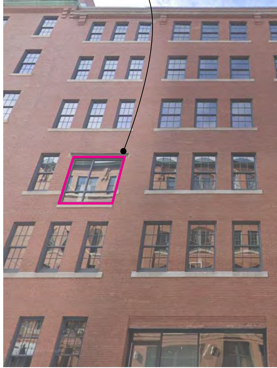
20 Channel Center - Channel Center Facade
