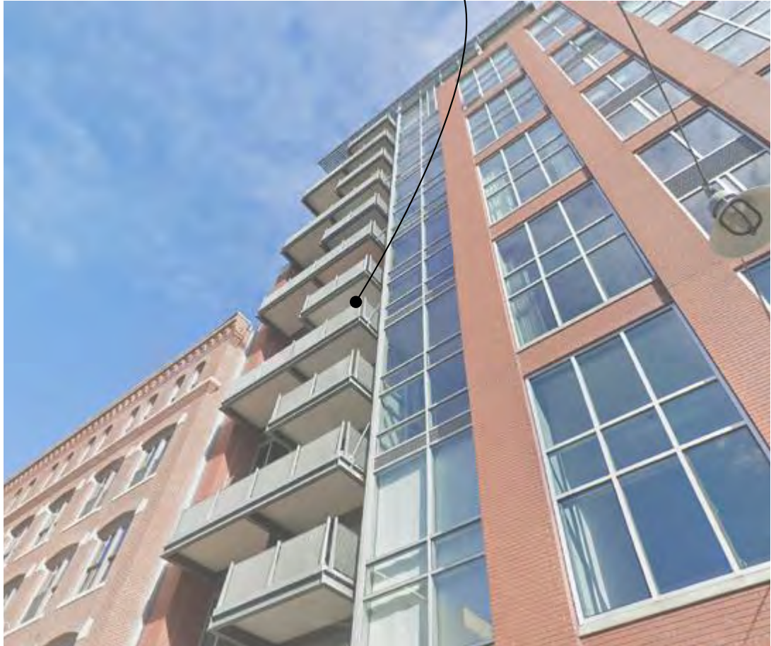
25 Channel Center - Channel Center Facade
