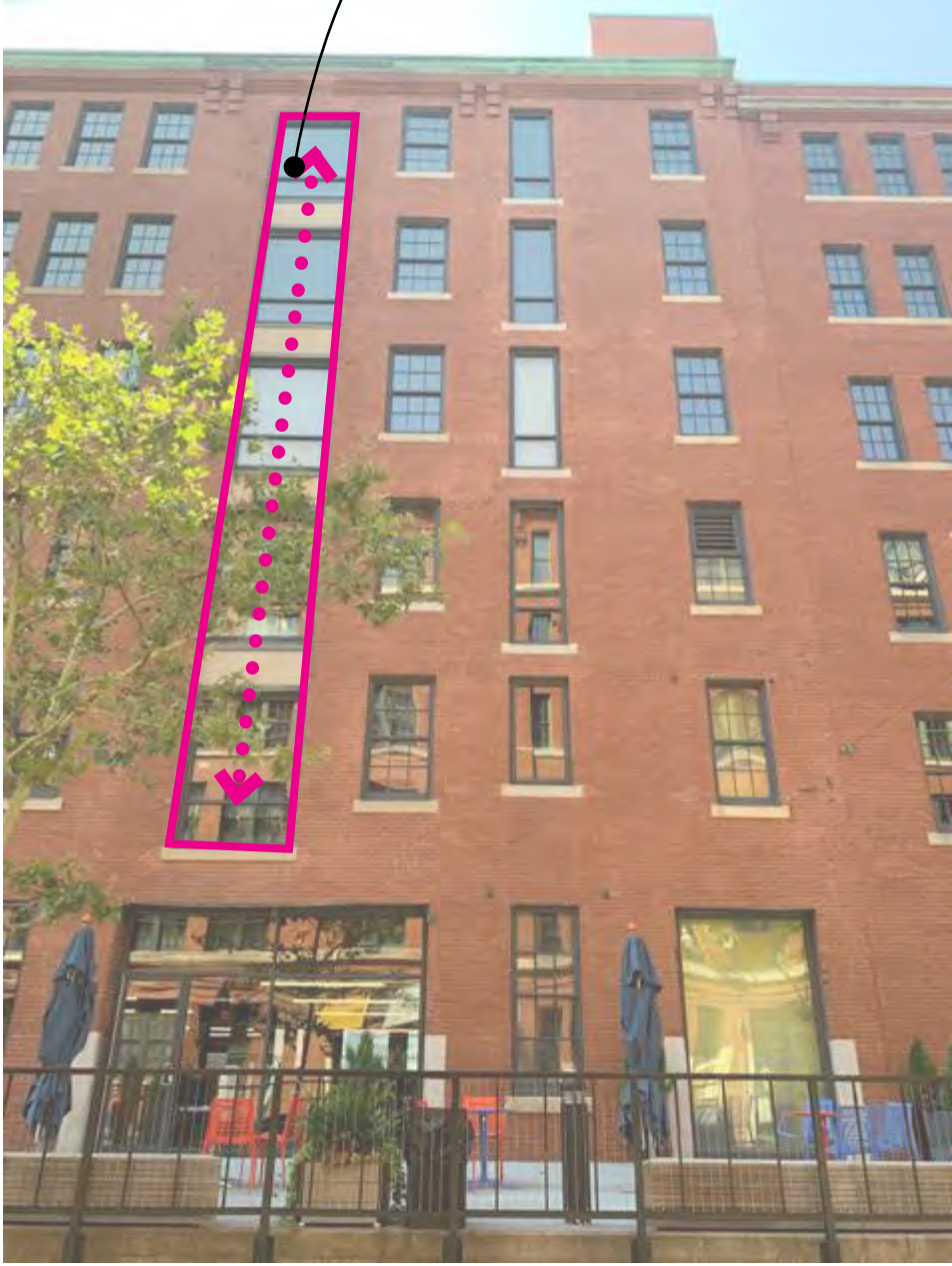
20 Channel Center - Channel Center Facade
