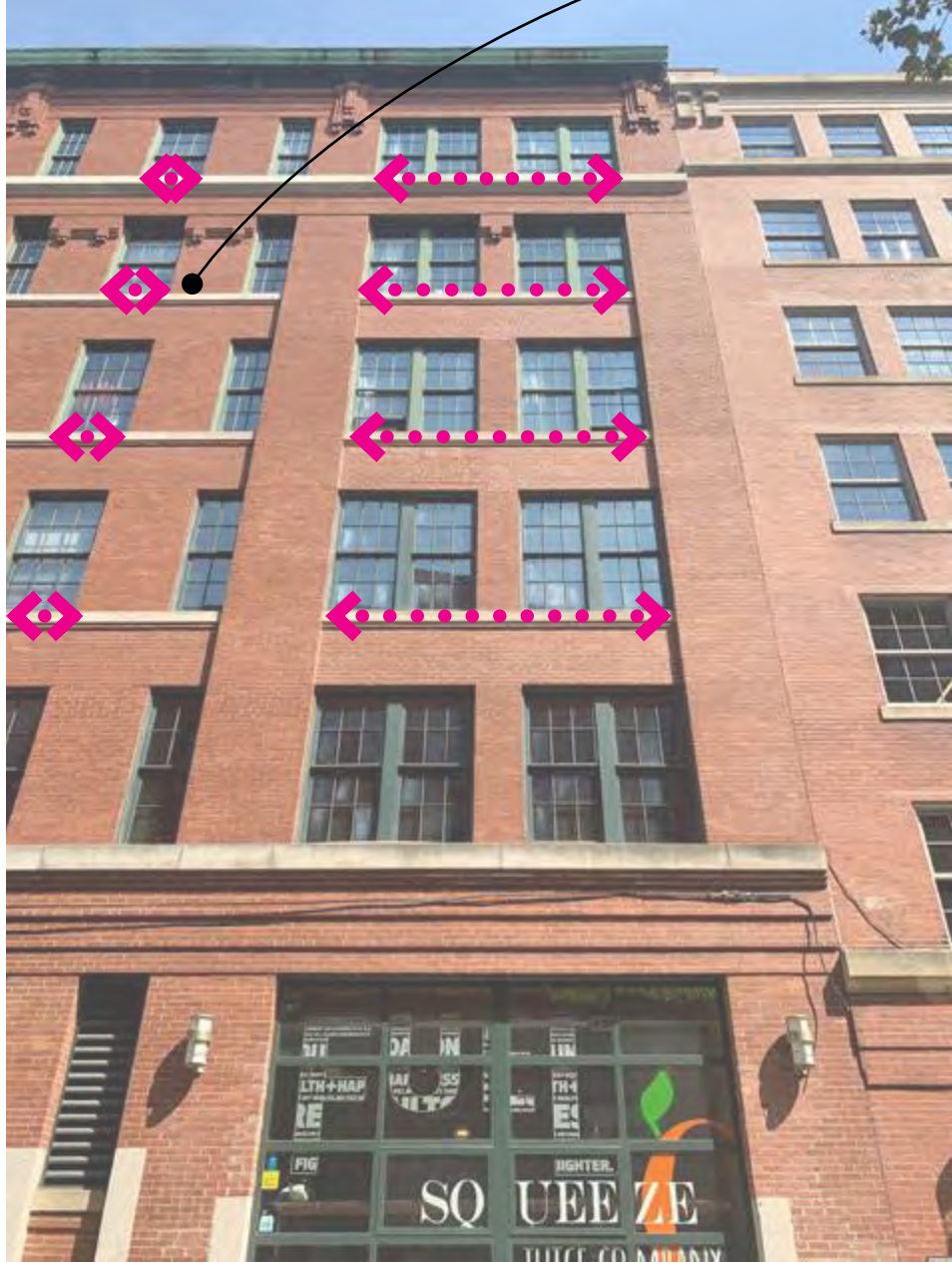
15 Channel Center - Channel Center Facade
