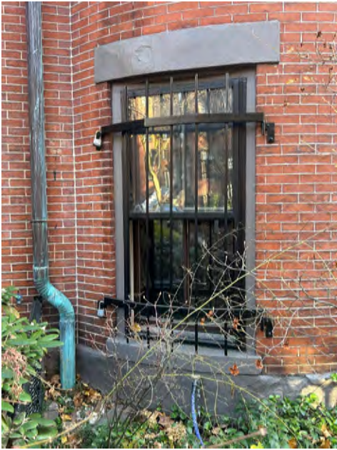
First floor window north
