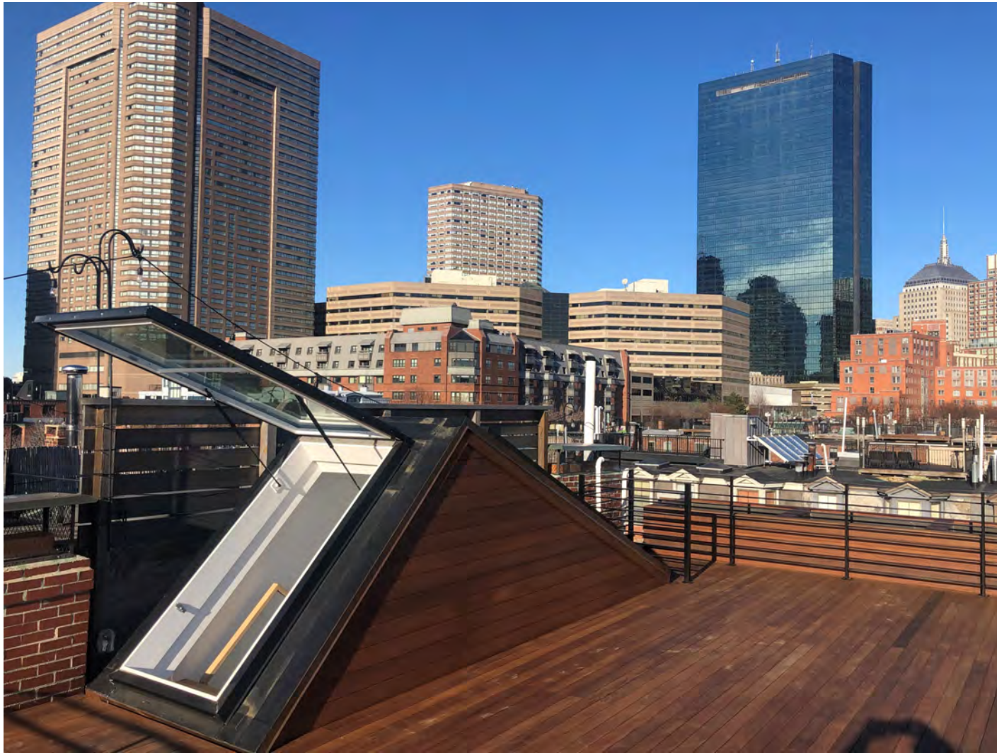
Roof deck access hatch example at 24 Holyoke.
