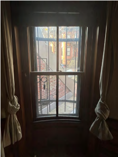
First floor window south interior
