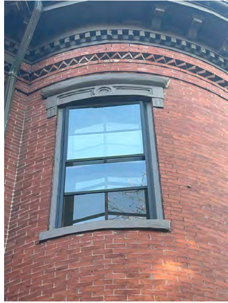
Third floor windows exterior
