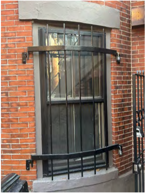
First floor windows south
