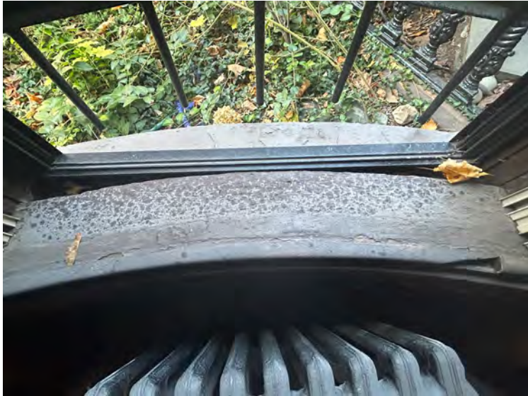
First window north interior
