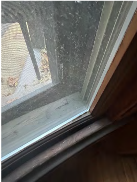
First floor windows showing Double glazing
