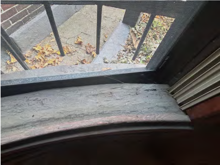
First floor window south interior
