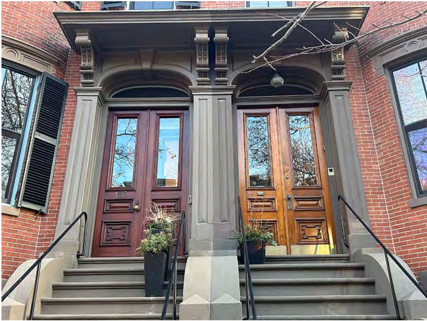
181 and 183 West Brookline with glazed door panels
