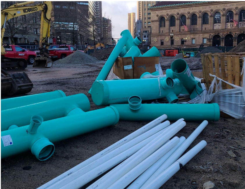
Drainage pipe awaits installation on site.
