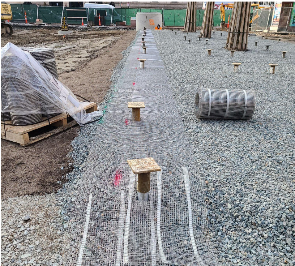
At the Raised Grove, we have now added planting soil, crushed stone, and stainless rodent mesh on top.
