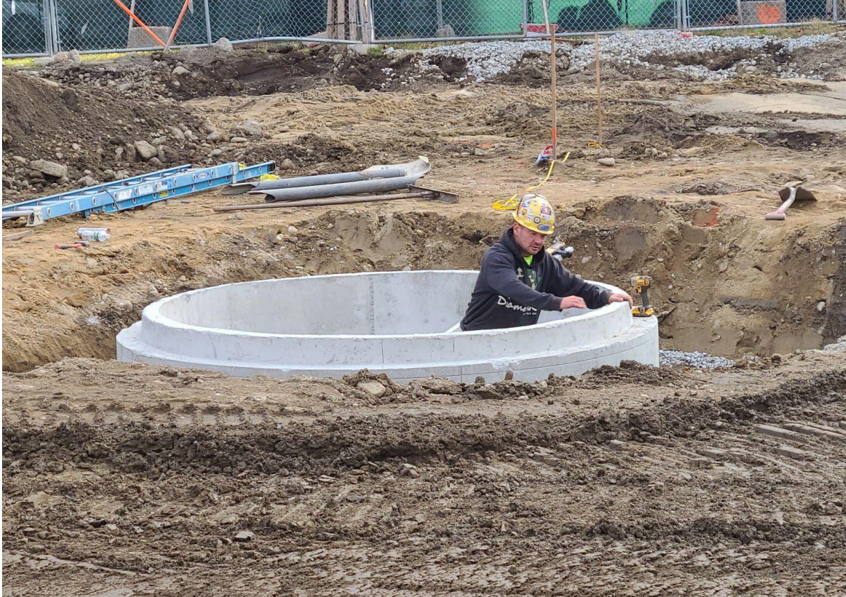
One of our larger drainage structures is being installed.
