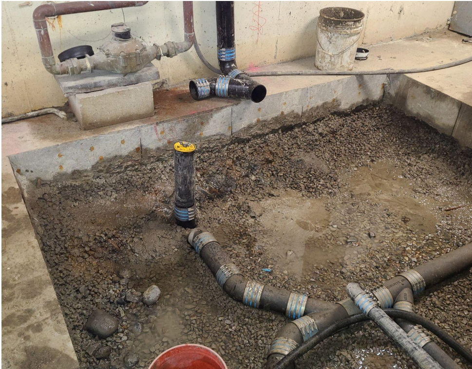
Modifying the drainage below the floor of the fountain vault.
