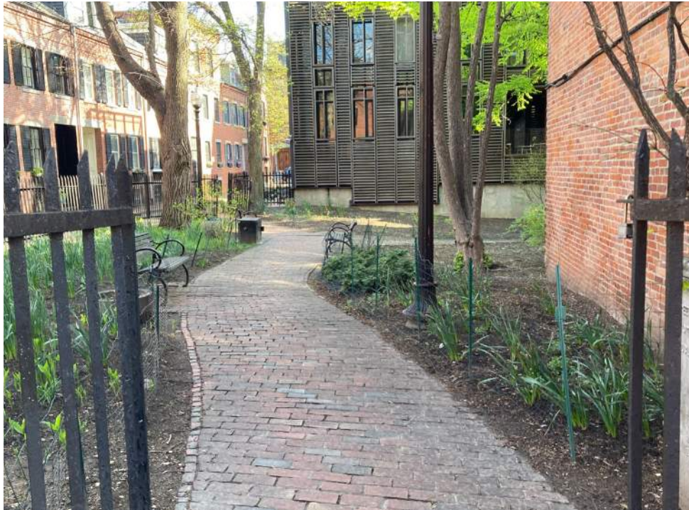
EXISTING PATHWAY LIMITS COMMUNITY GATHERING AND HAS AN INACCESSIBLE CROSS PITCH.
