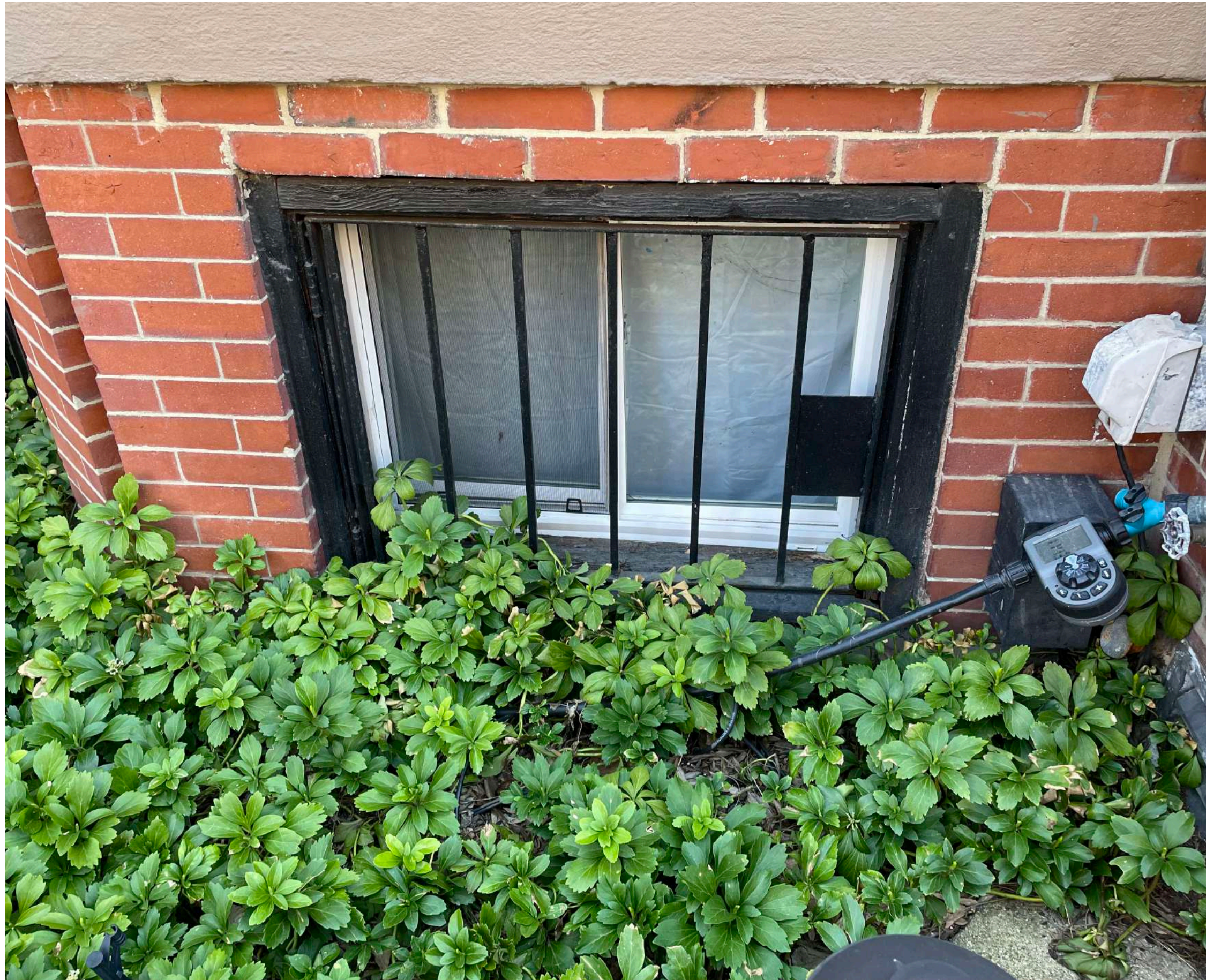
GARDEN LEVEL WINDOW @332 SHAWMUT
