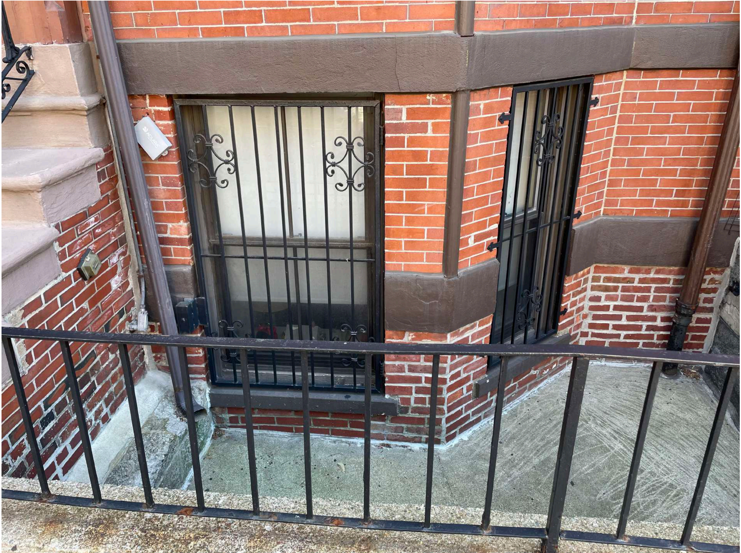
334 SHAWMUT AVE GARDEN LEVEL WINDOWS
