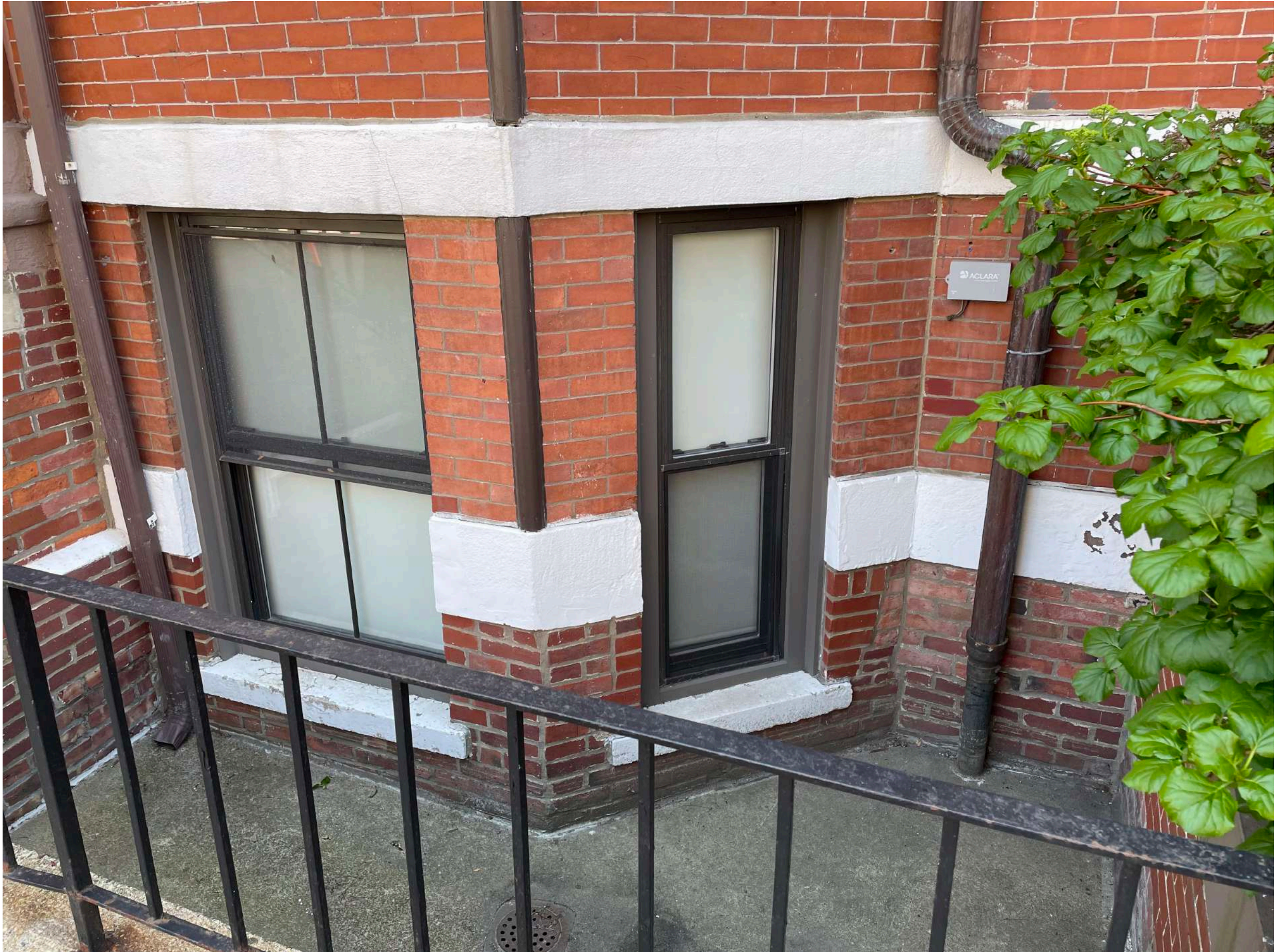
#330 SHAWMUT AVE GARDEN LEVEL WINDOWS
