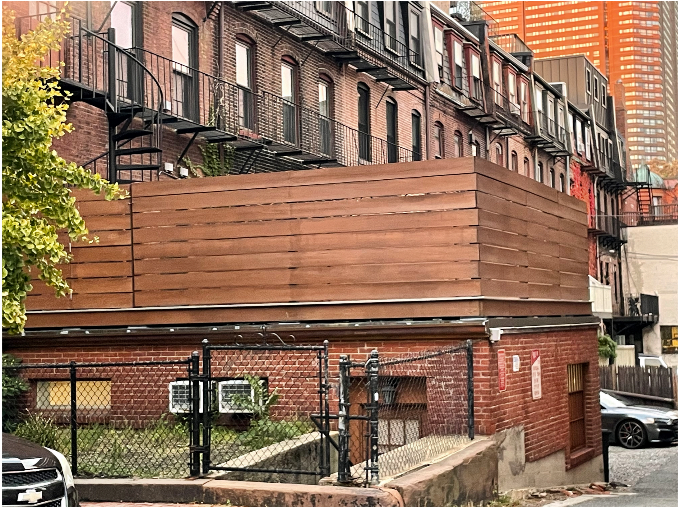
116 St. Botolph Street - Durham Street front and side alley
