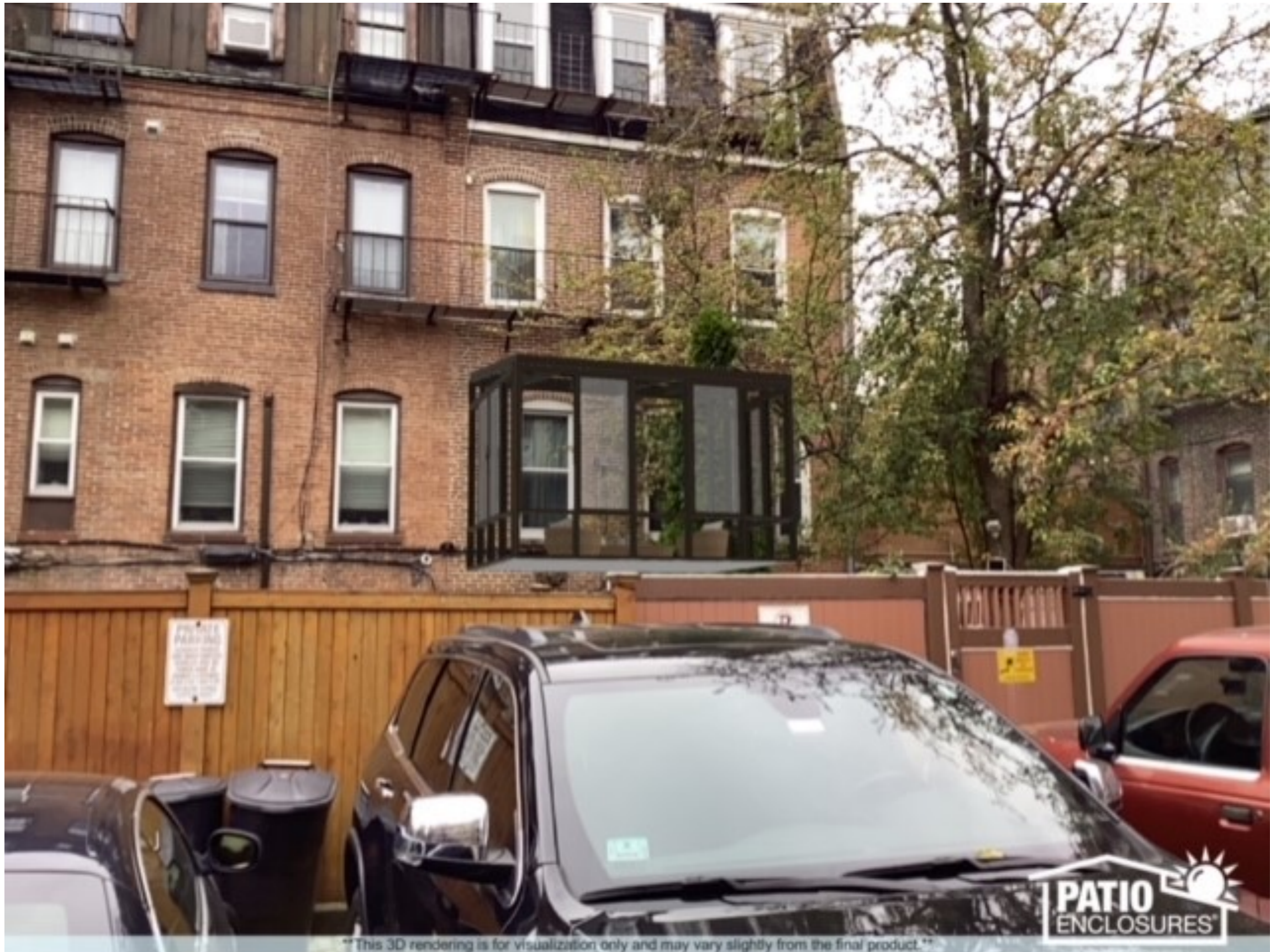
2 Durham Street with Addition
