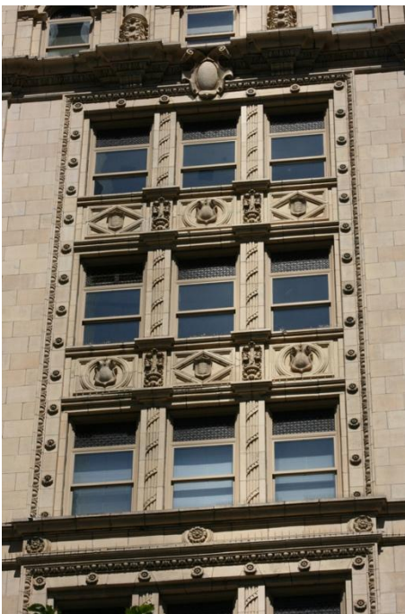
Figure 7. Washington Street façade, detail of floors 6, 7, and 8.
