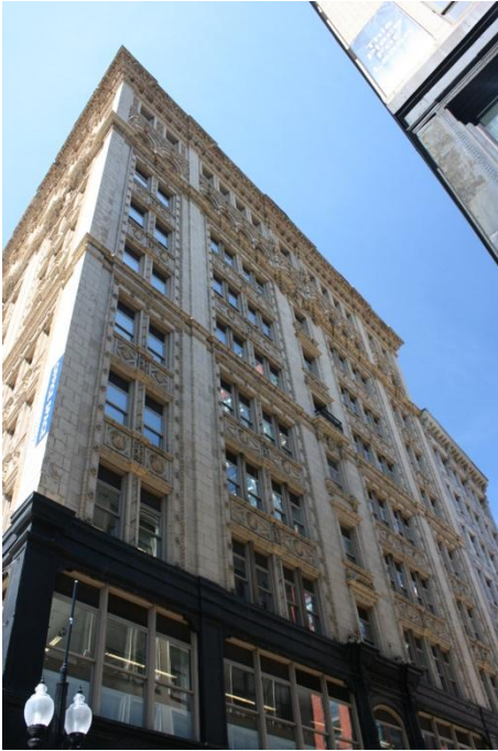
Figure 4. Bromfield Street (north) façade.
