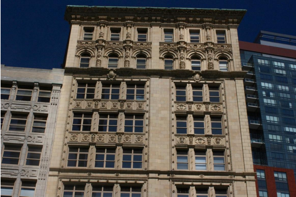
Figure 6. Washington Street façade, floors 6 through 10.
