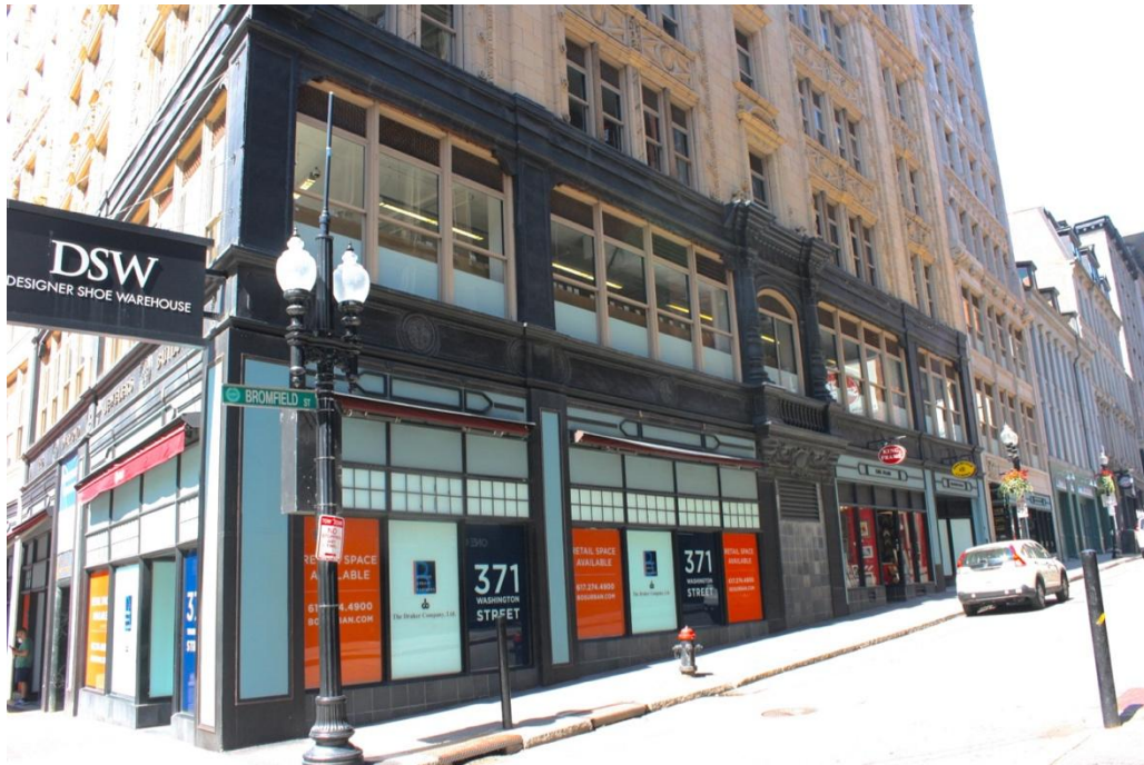
Figure 5. Bromfield Street facade, storefronts.
