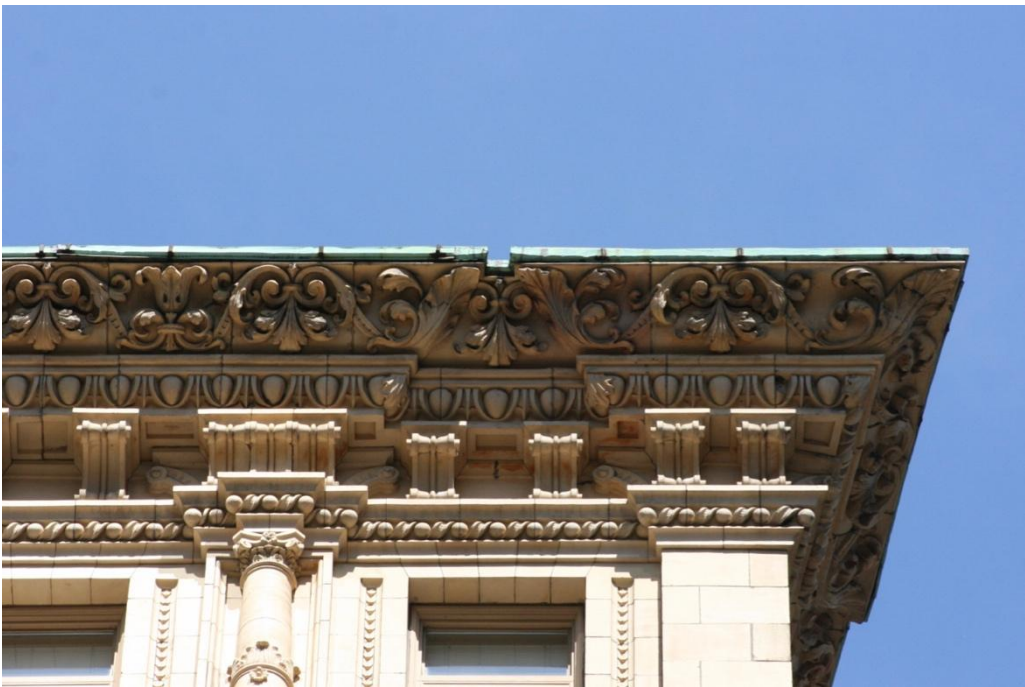
Figure 9. Washington Street elevation; detail of cornice.
