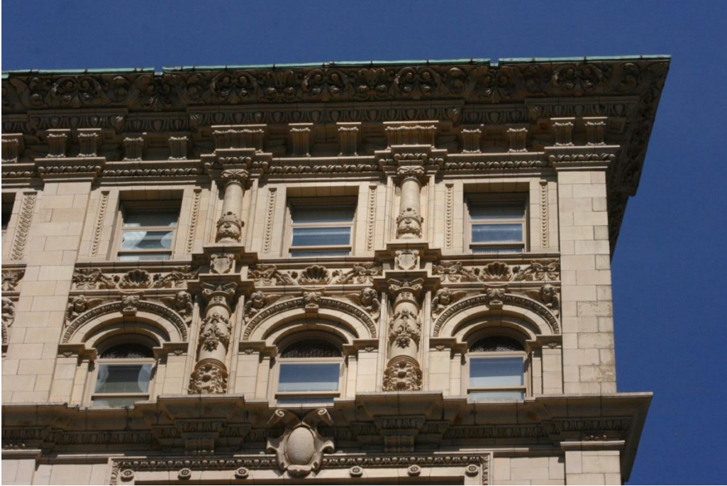
Figure 8. Washington Street elevation, detail of floors 9 and 10.
