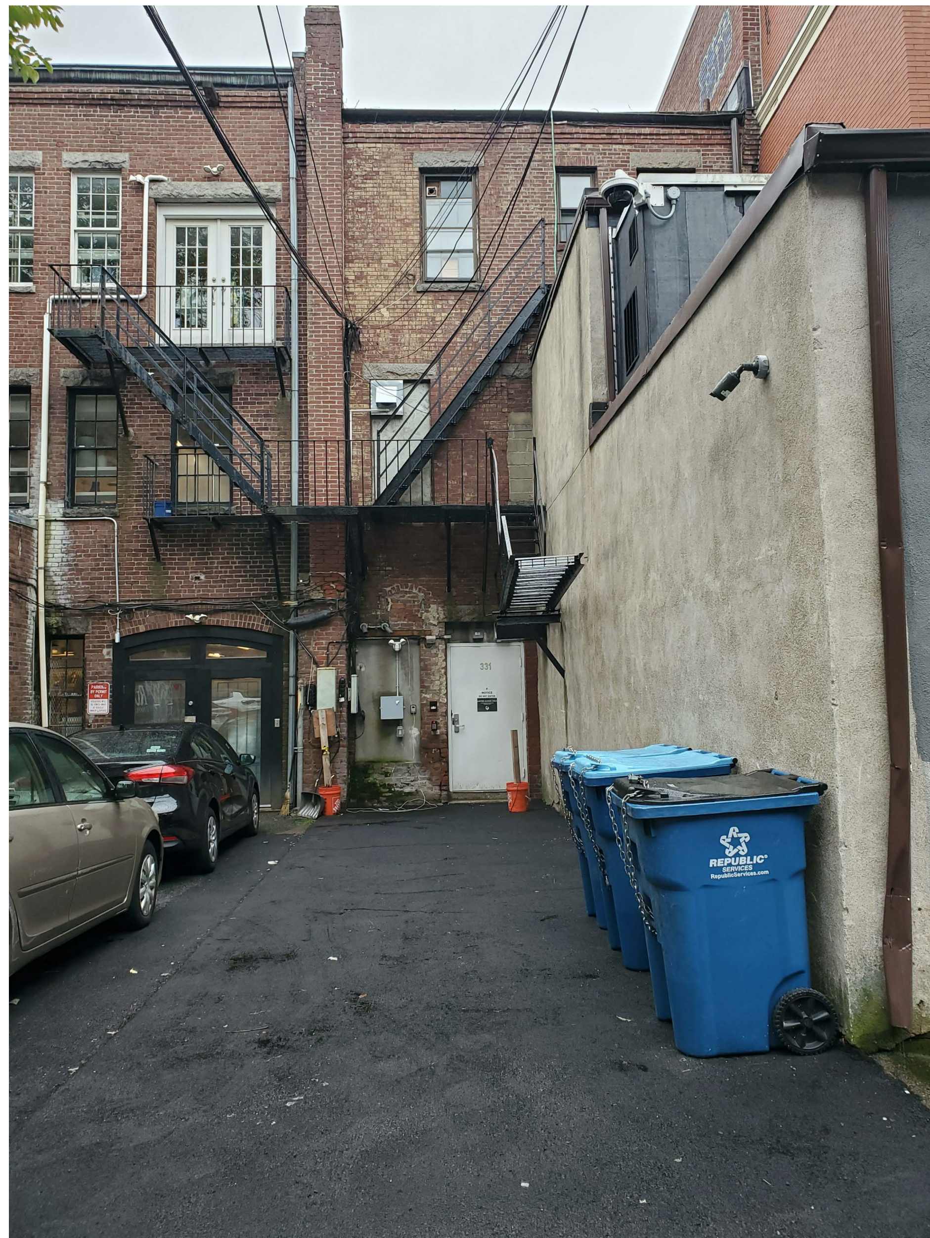
EXISTING REAR FACADE VIEW FROM ALLEY
