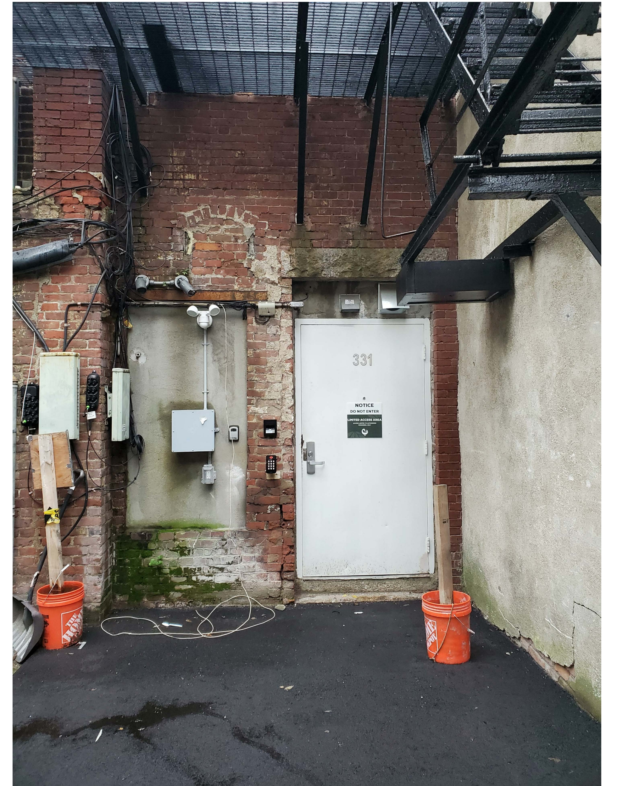
EXISTING REAR ENTRY
