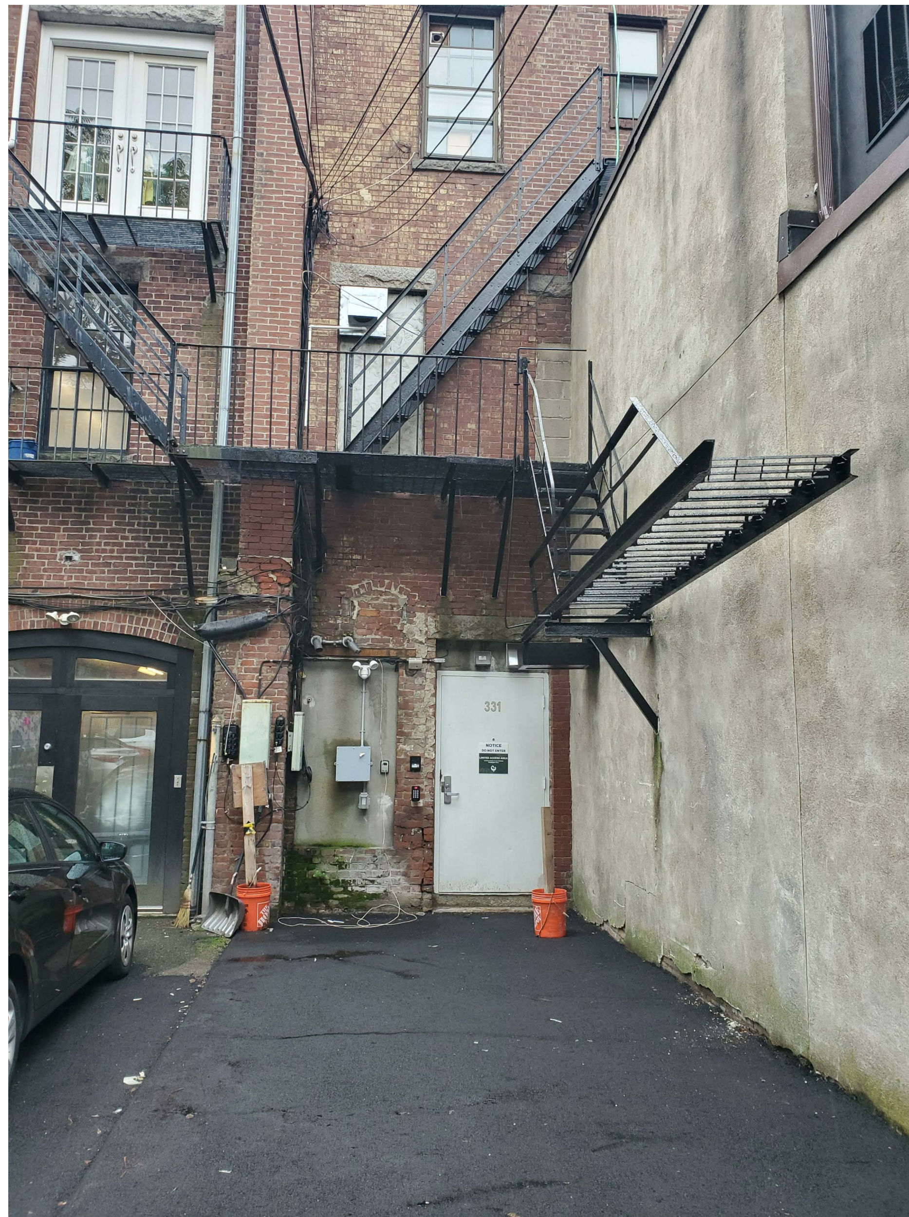
EXISTING REAR FACADE VIEW FROM PARKING
