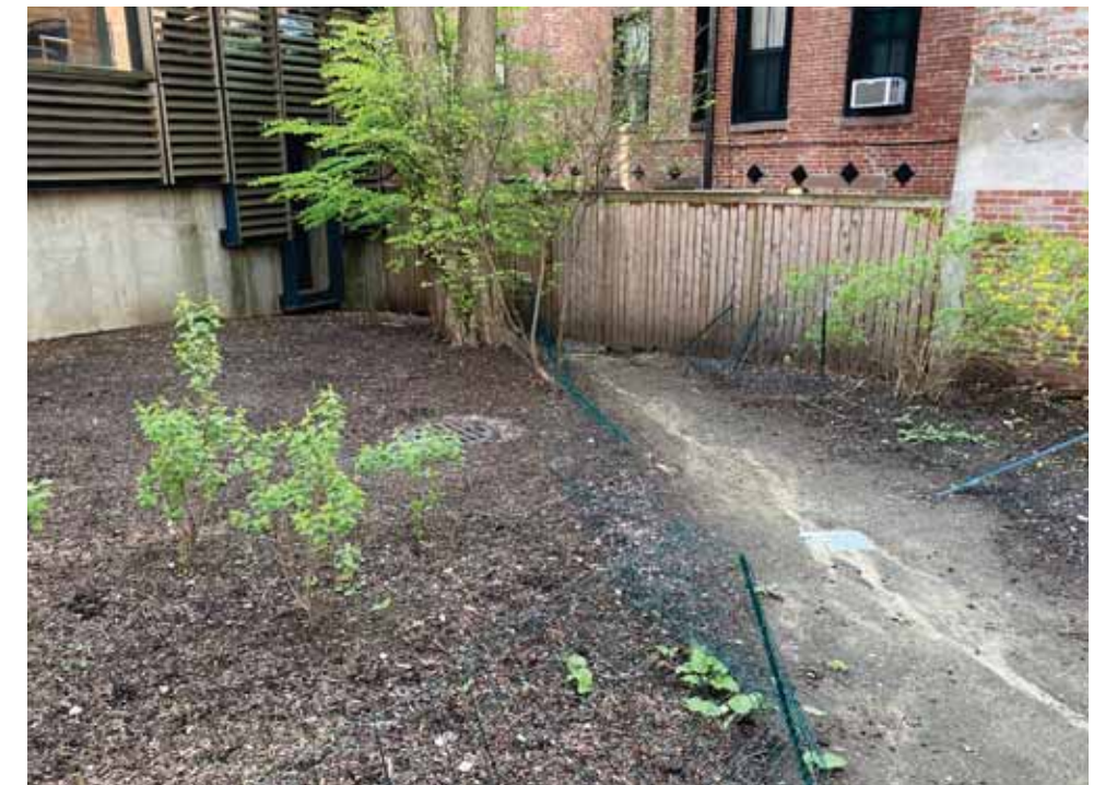
SLOPED GRADE ACROSS WATSON PARK CHANNELS STORM WATER INTO THE ADJACENT PROPERTY.
