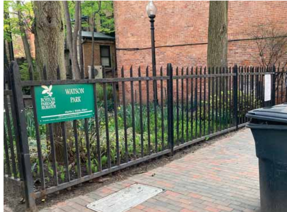
TALL PERIMETER FENCING IS NOT INVITING AND EXCLUDES TAYLOR ST. FROM THE PARK EXPERIENCE.
