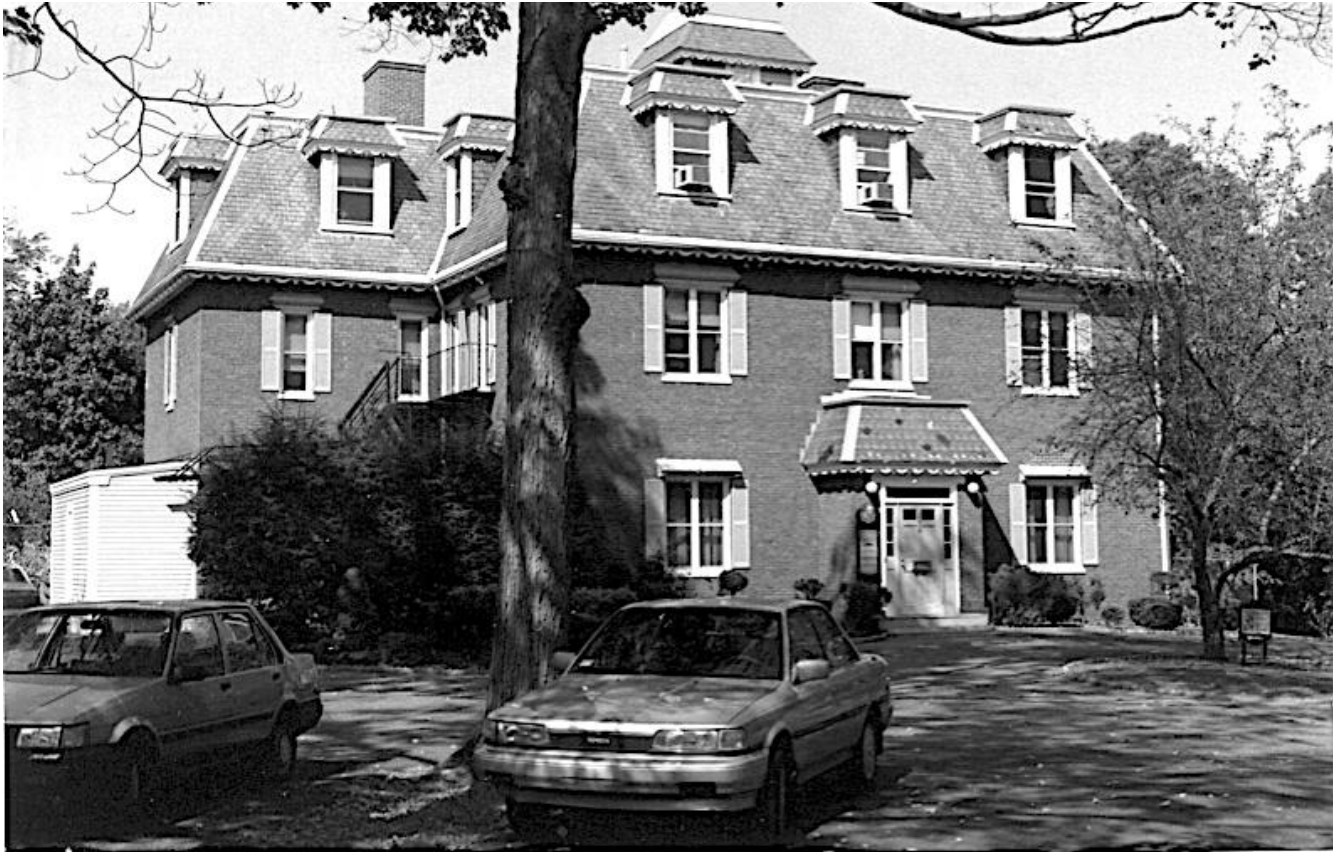
Figure 23. View of façade, looking northeast, ca. 1977.
