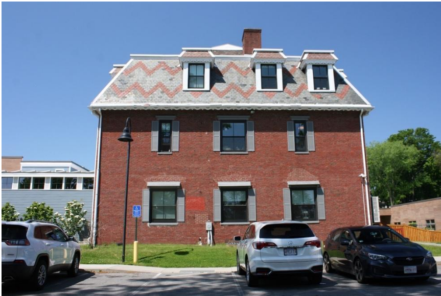
Figure 11. East elevation. Photograph by Wendy Frontiero, June 2023.
