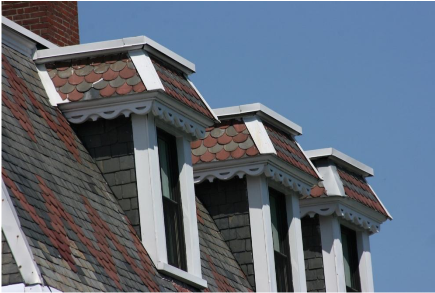
Figure 14. Detail of dormers. Photograph by Wendy Frontiero, June 2023.
