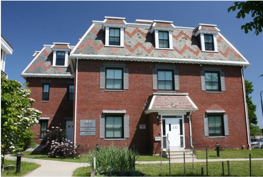
Figure 4. Façade (south elevation). Photograph by Wendy Frontiero, June 2023.
