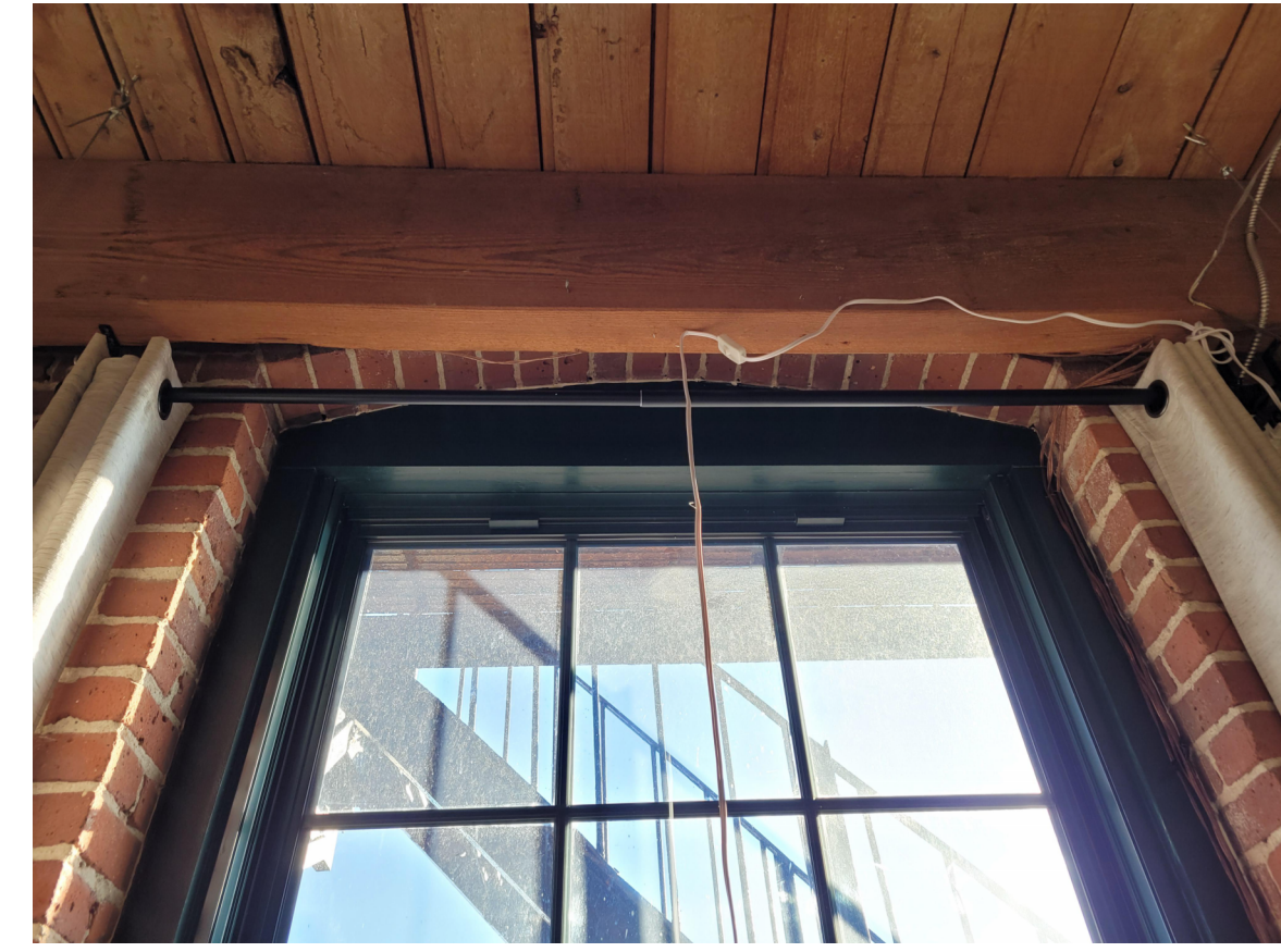
EXISTING SEGMENTAL ARCH ON INTERIOR SIDE
