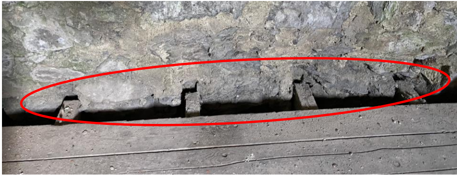
ROTTING JOIST ENDS
