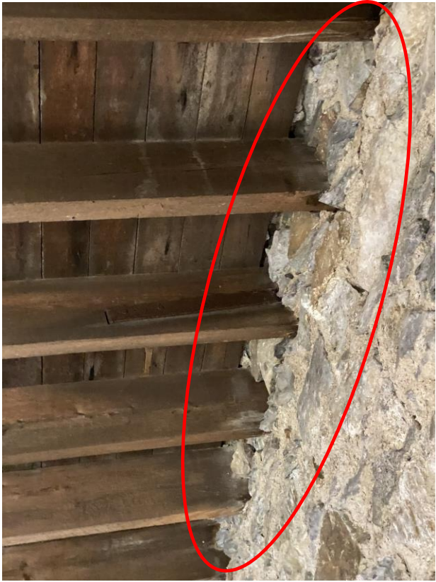
ROTTING JOIST ENDS
