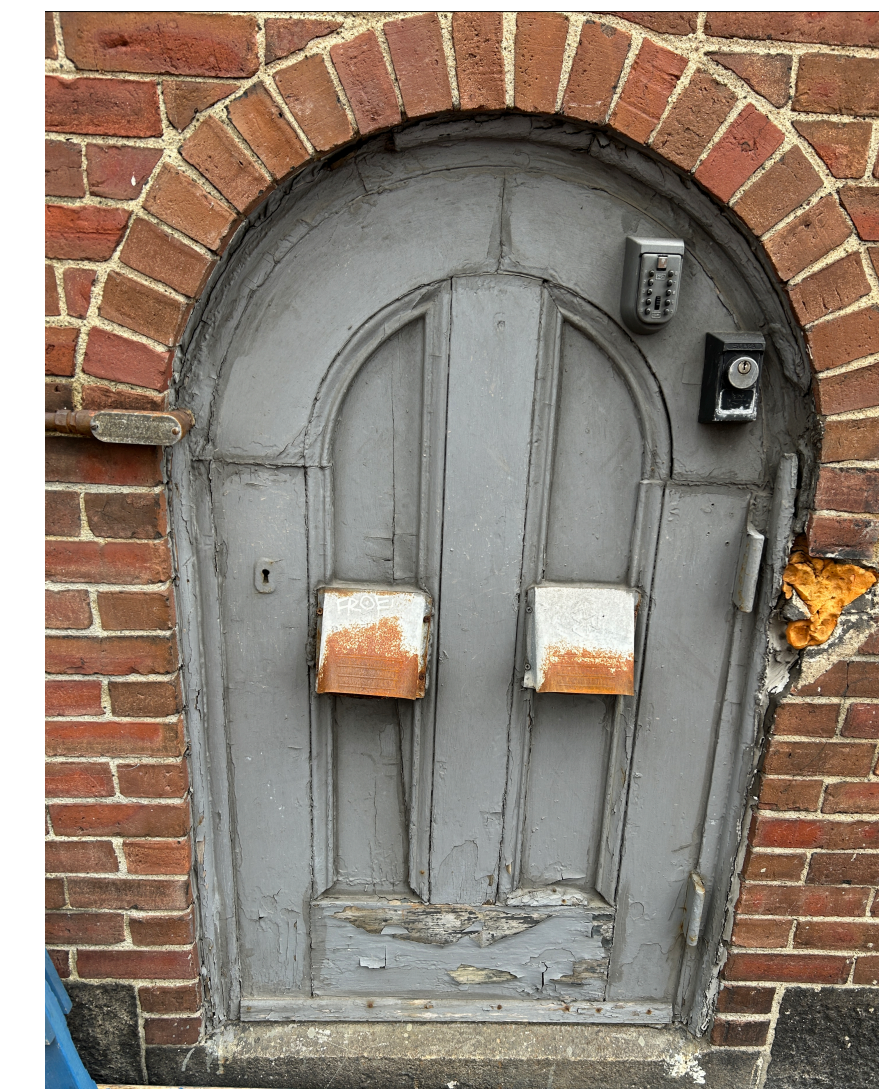
2 OTIS PLACE EXISTING DOOR ON MT.VERNON STREET PROVIDING CONTEXTUAL RELEVANCY FOR PROPOSING DOOR AT 1 OTIS. PANEL ARRANGEMENT TO INFLUENCE ADJACENT ARCHED DOOR AT 1 OTIS
