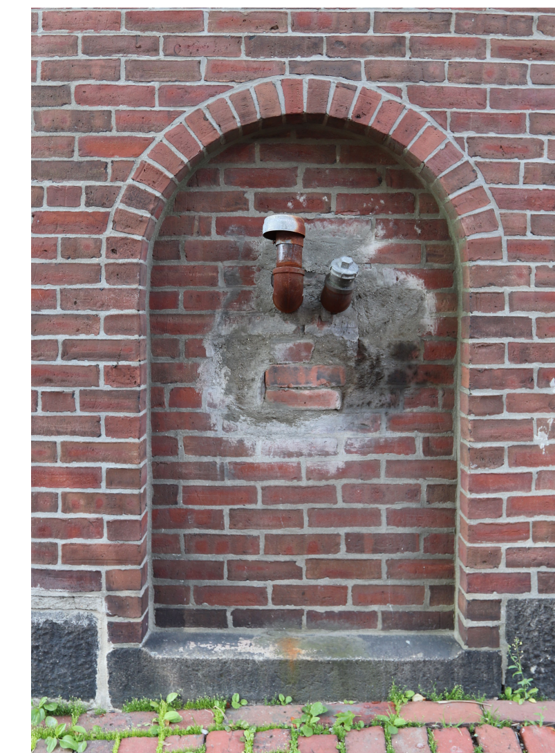
1 OTIS PLACE EXISTING ARCHED PARTIAL OPENING ON MT.VERNON STREET TO BECOME A FULL OPENING WITH A WOOD, BI-FOLD DOOR W/MOLDING PROFILES TO MATCH ADJACENT FULL HEIGHT DOOR
