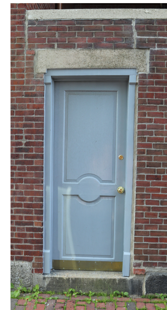
1 OTIS PLACE EXISTING GARDEN WALL DOOR ON MT.VERNON ST. TO BE REPLACED BY 4-PANEL WOOD DOOR W/BOLECTION MOLDING PROFILE TO MATCH DOORS THROUGHOUT HOUSE
