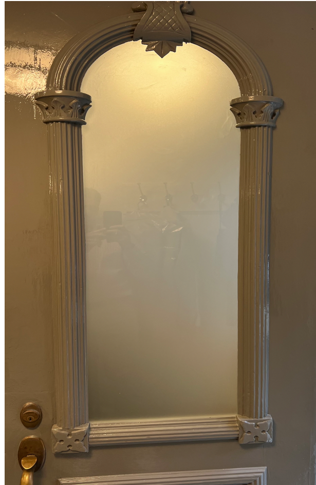
Repaired Widows- closeup
