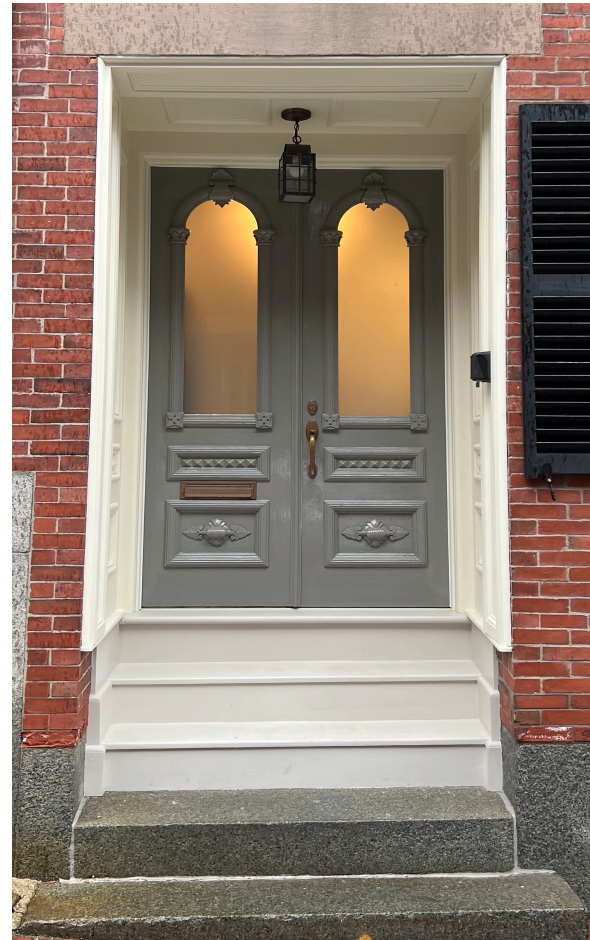
Repaired and Proposed Permanent
