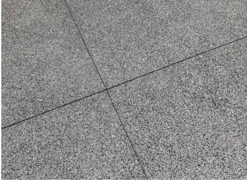
Proposed Exposed Aggregate Concrete Sidewalk
