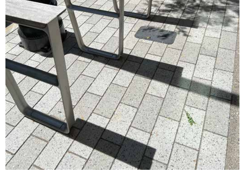
Proposed Permeable Concrete Unit Pavers
