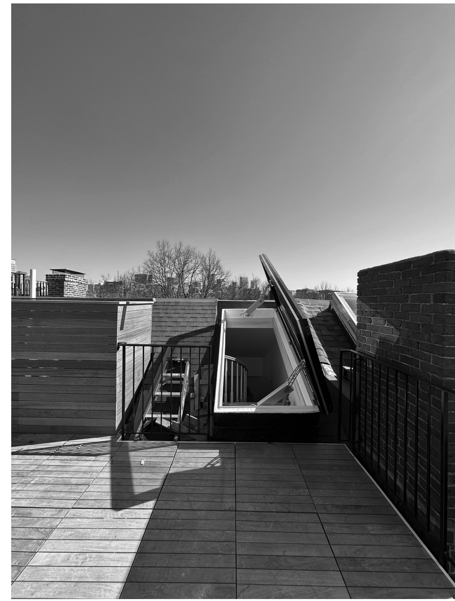
2 ROOF EXIT HATCH IN SITU
