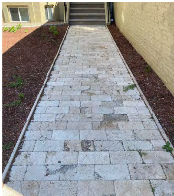
1615 Tremont St – Front Walkway
