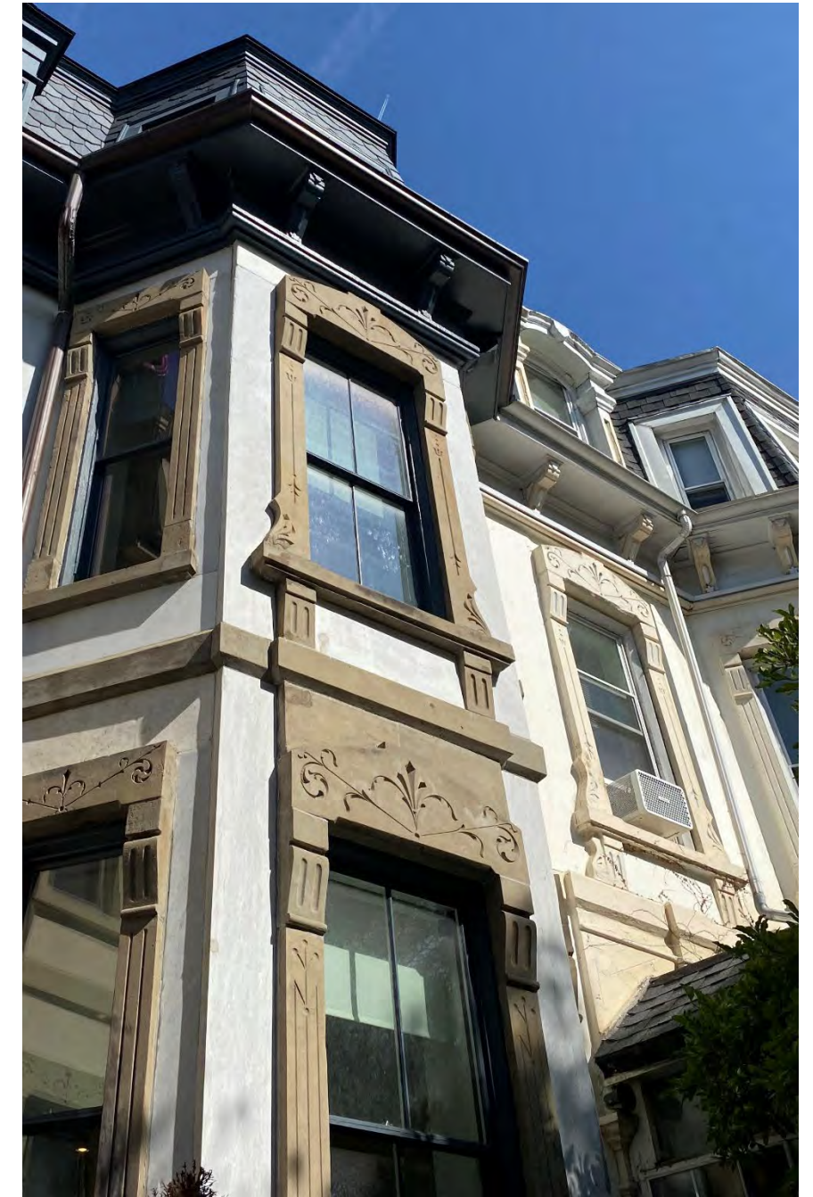
Stone Detail Precedent 1607 Tremont Street
