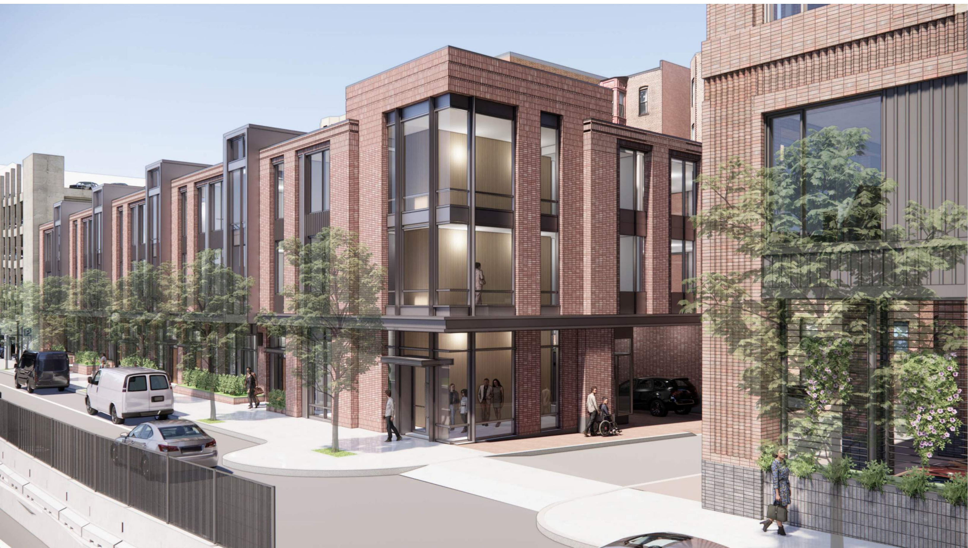
3-STORY BUILDING SOUTHEAST CORNER
