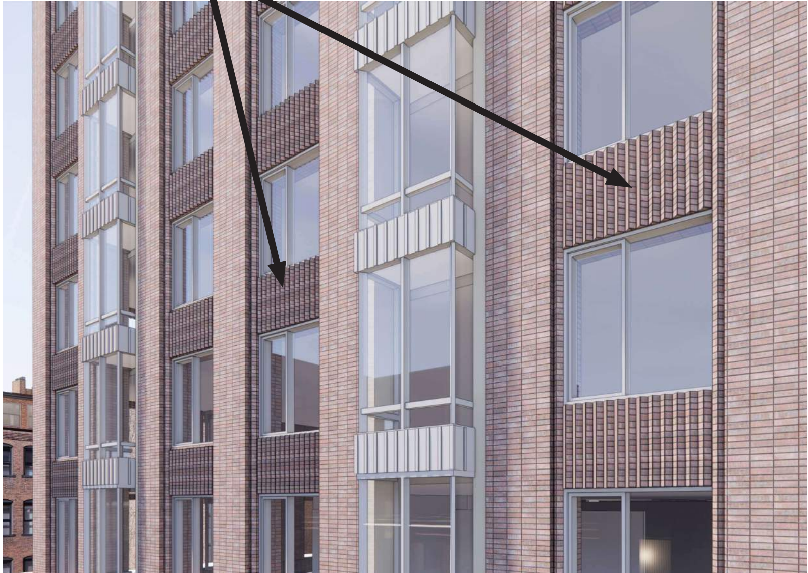
PROPOSED MASONRY DETAILING
