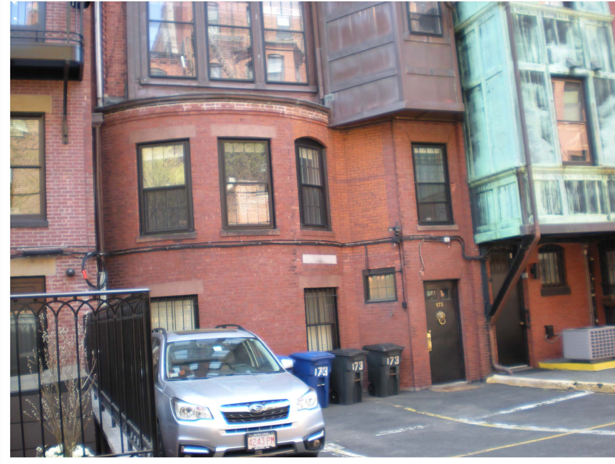
② MASONRY BAY VIEW FROM EAST
