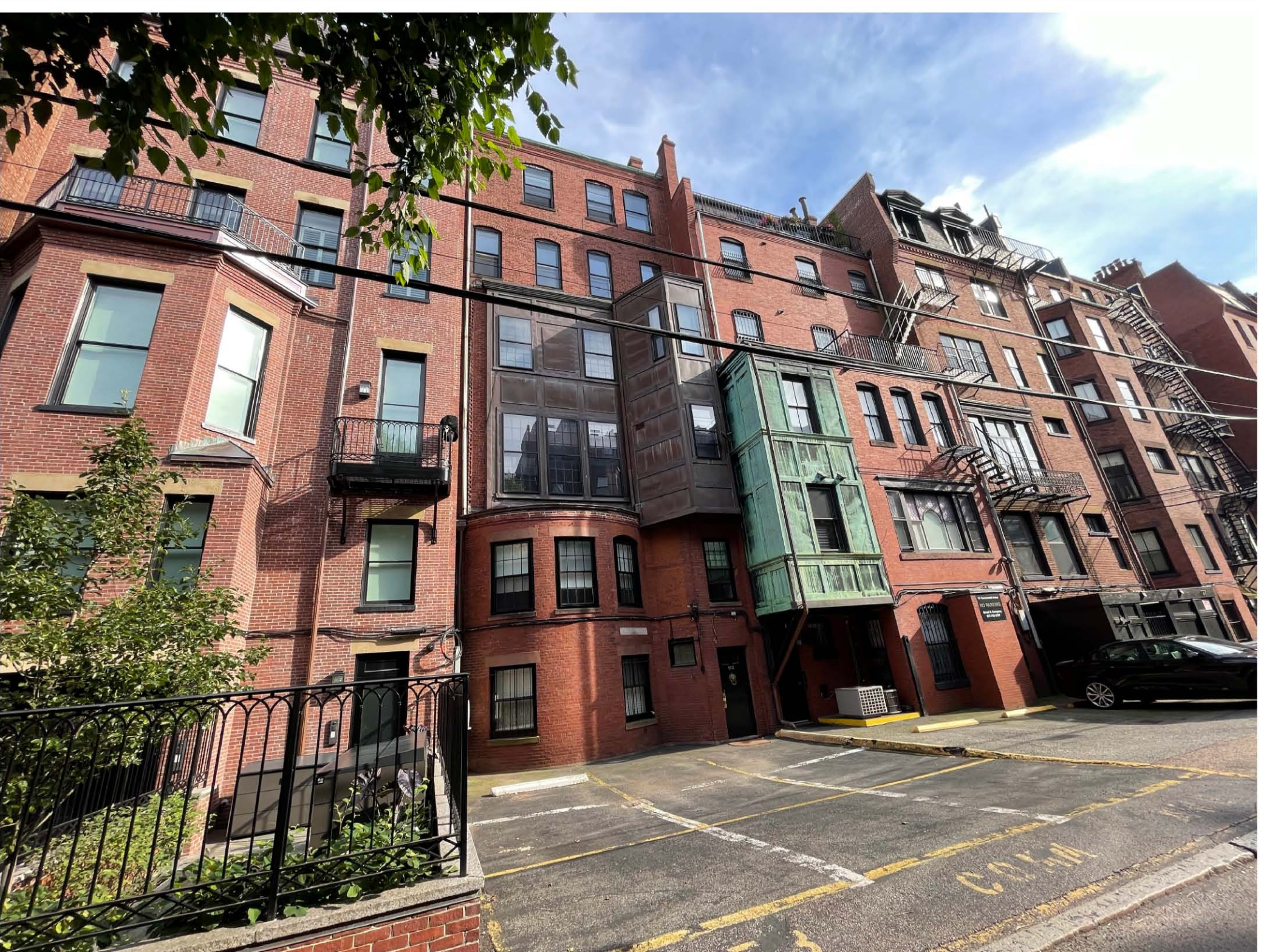
④ REAR FACADE VIEW FROM EAST
