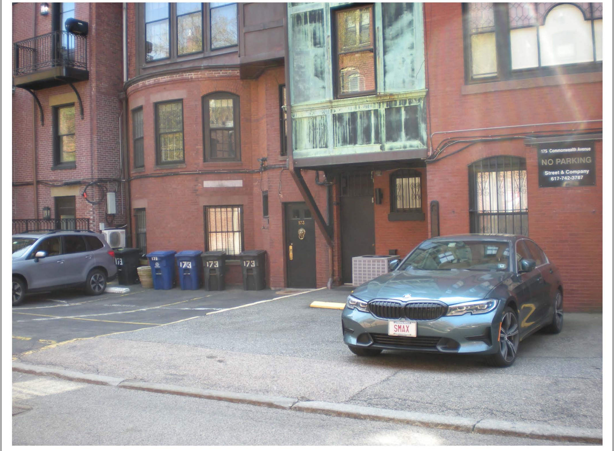
③ MASONRY BAY VIEW FROM WEST
