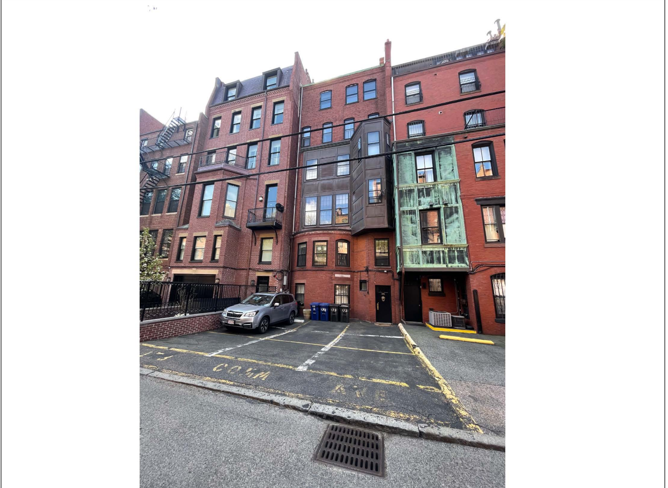
⑥ REAR FACADE VIEW FROM WEST
