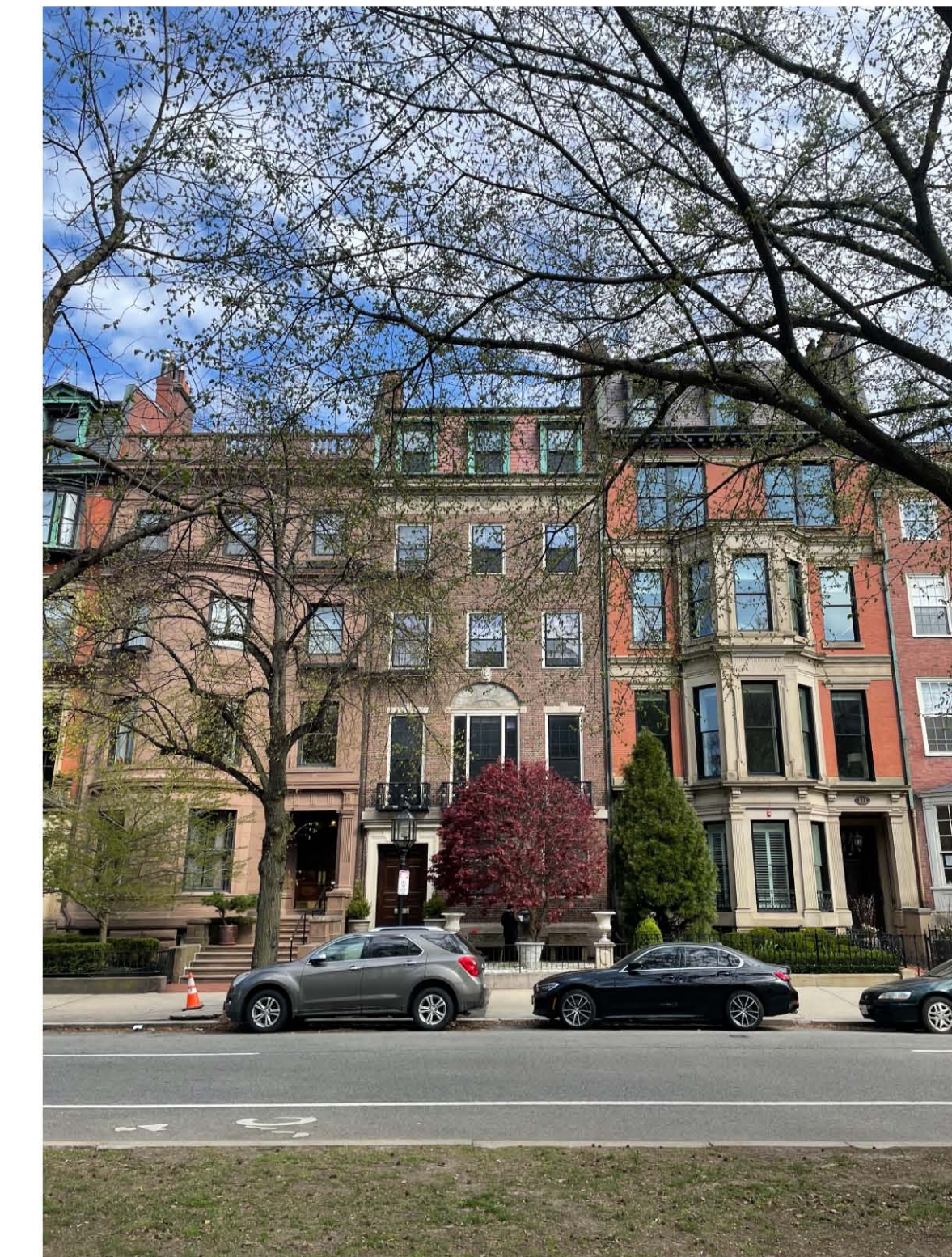
⑥ FRONT FACADE FROM COMMONWEALTH MALL
