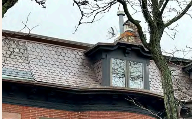
Composite mansard shingle restoration at 103 Warren Ave.
