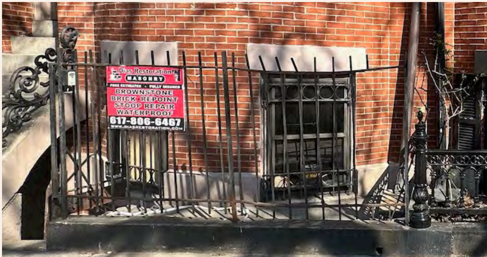
Existing Condition at 121 Warren Ave.
