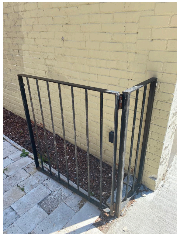
1615 Tremont St – Front Fence & Gate 1.1
