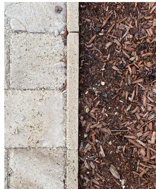
1615 Tremont St – Yard Materials
