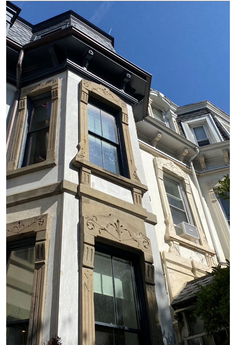
Stone Detail Precedent 1607 Tremont Street
