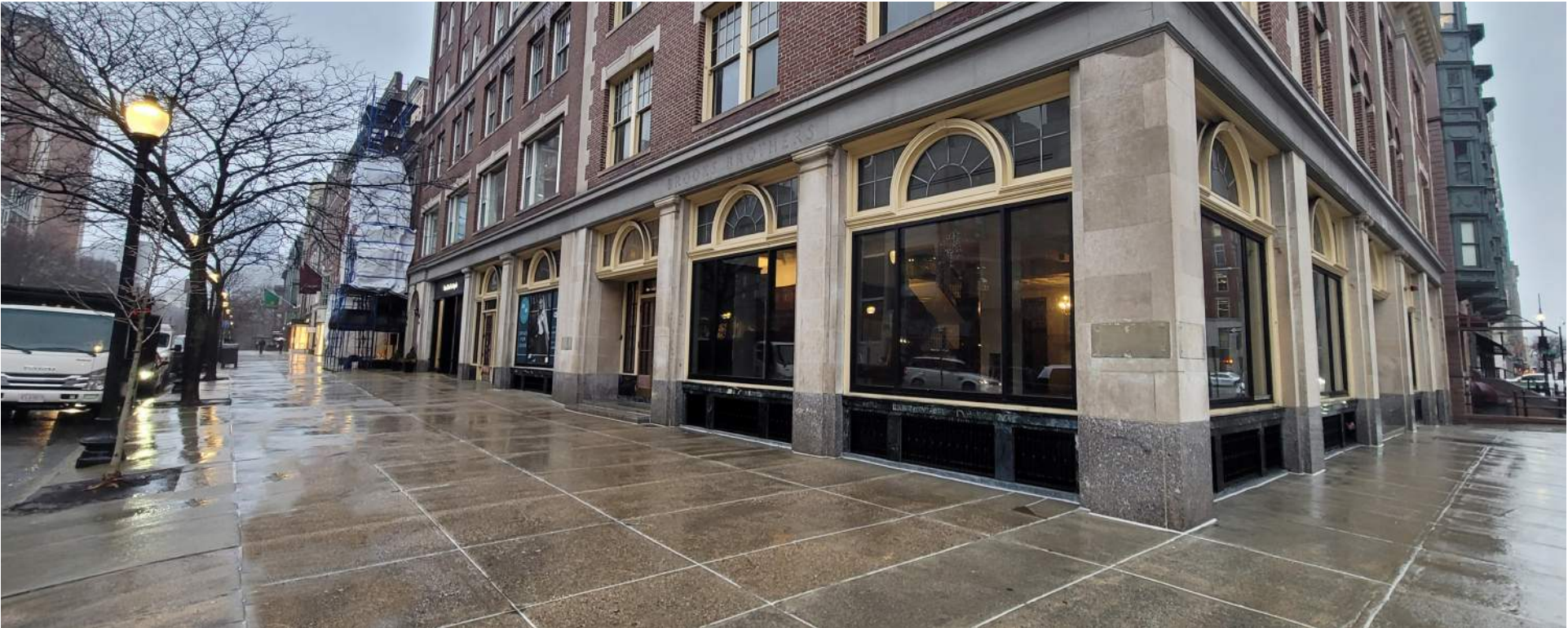
Existing Condition Photo
