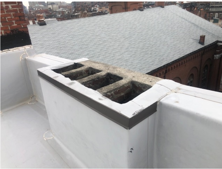
VIEW OF EAST FACING PERIMETER CHIMNEYS FROM ROOF
