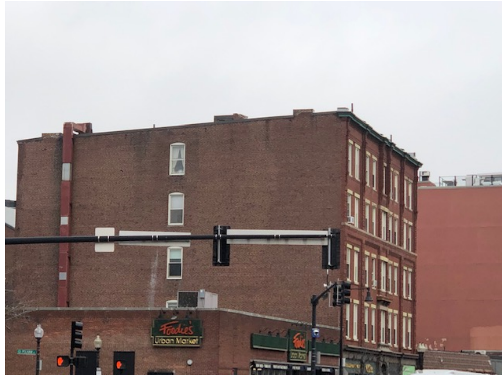
VIEW OF WEST FACING PERIMETER CHIMNEYS FROM WASHINGTON STREET
