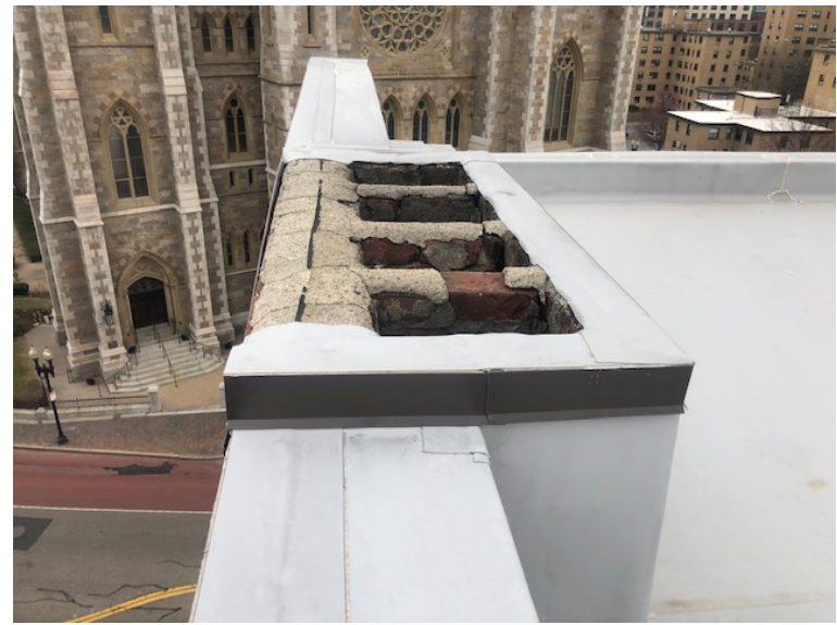
VIEW OF EAST FACING PERIMETER CHIMNEYS FROM ROOF
