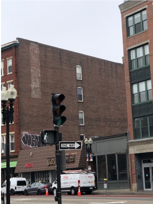
VIEW OF EAST FACING PERIMETER CHIMNEYS FROM THE SE
