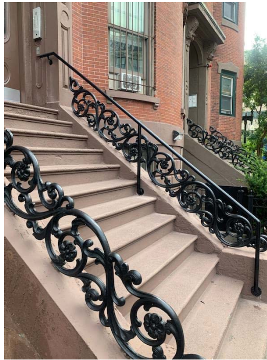
Posts Tied into Stringer 698 Mass Avenue
