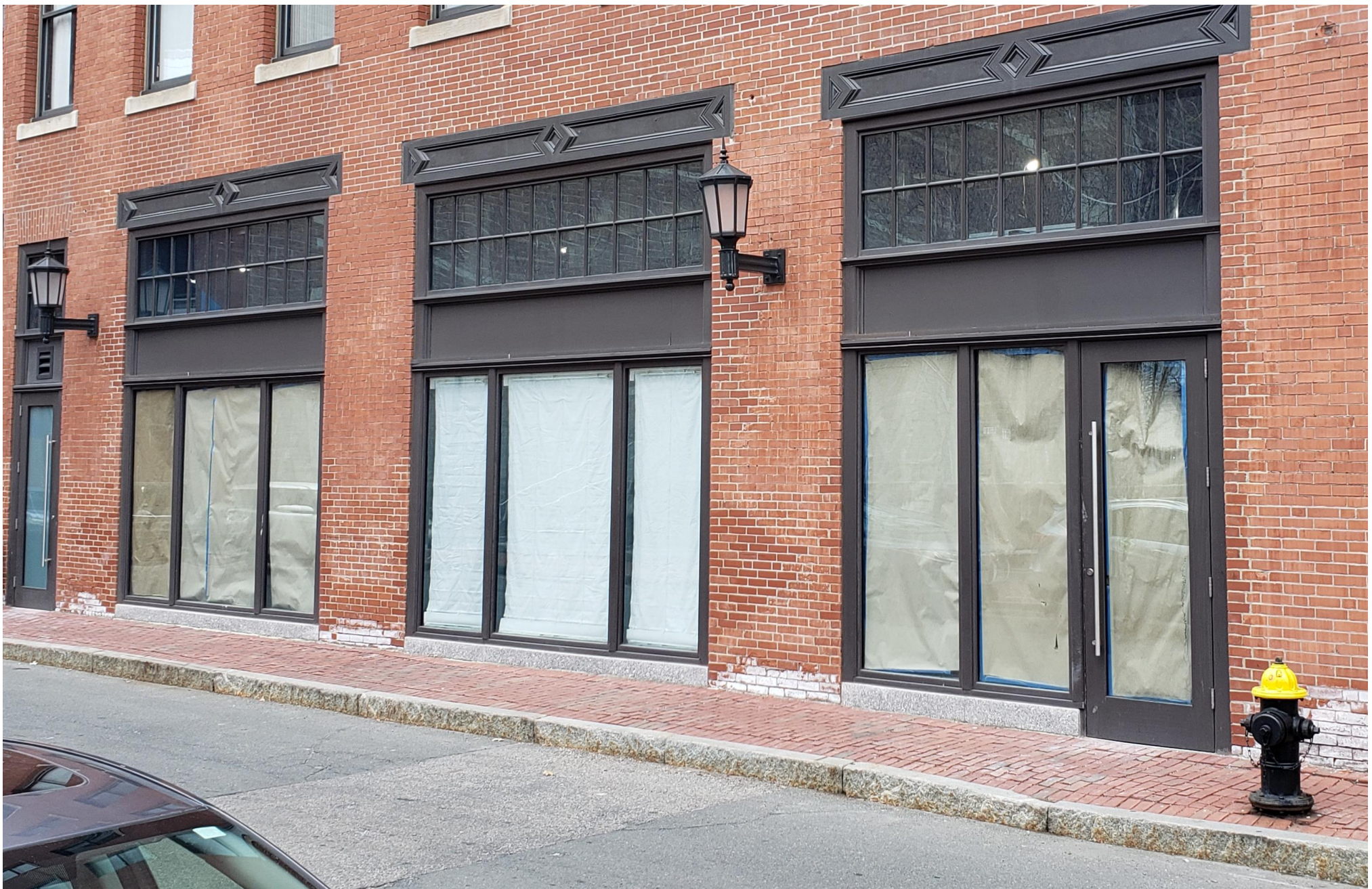
EXISTING CONDITION PHOTO
