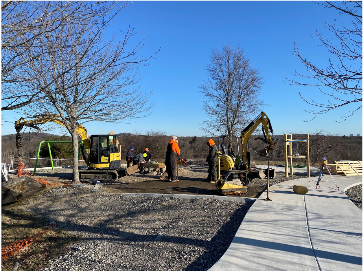
2-5 play area under construction
