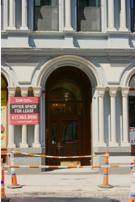
Figure 8. State Street façade; detail of main entrance.
