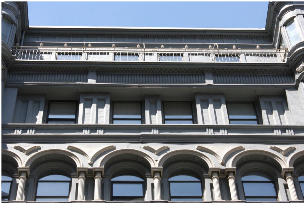
Figure 5. State Street façade; detail of 6th and 7th floors.
