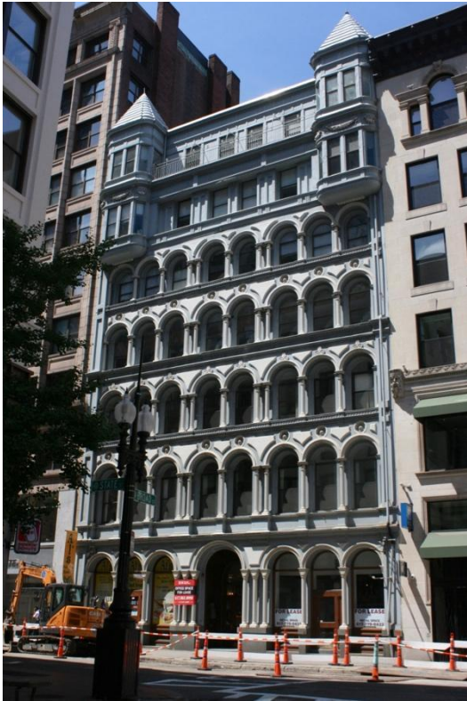
Figure 2. State Street façade.
