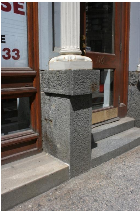
Figure 7. State Street façade; detail of column base at ground floor.
