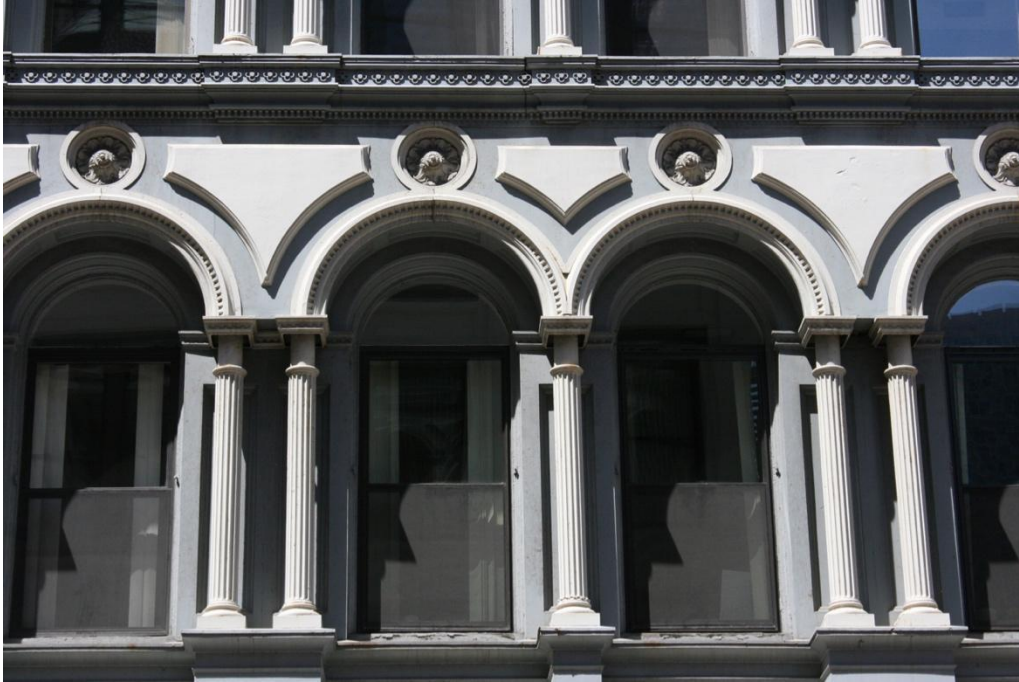
Figure 12. State Street façade; detail of second-floor arcade.
