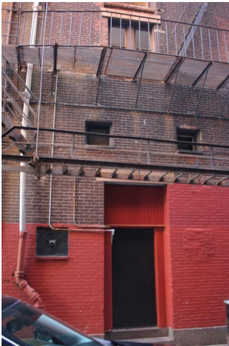
Figure 17. Butler Square elevation; center entry.
