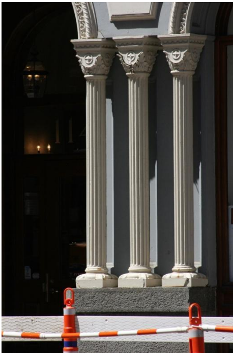
Figure 9. State Street façade; detail of columns at main entrance.
