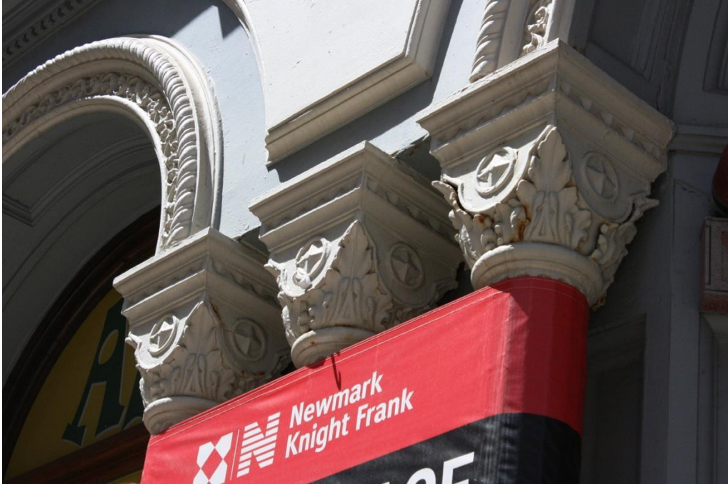
Figure 10. State Street façade; detail of column capitals at main entrance.
