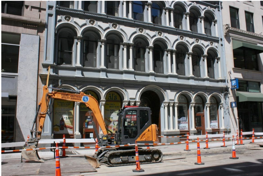
Figure 4. State Street façade; detail of 1st and 2nd floors.
