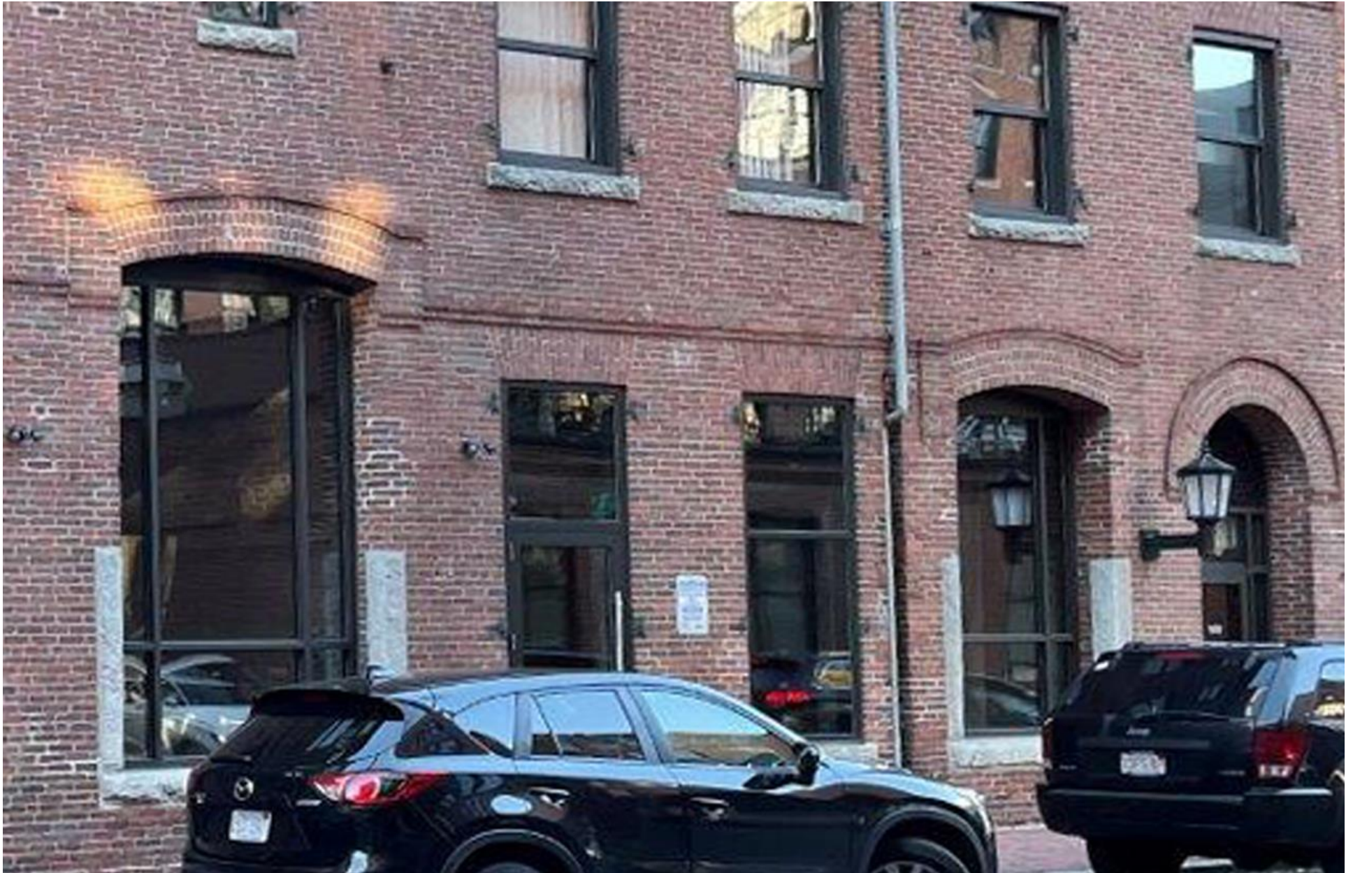
EXISTING CONDITION PHOTO
