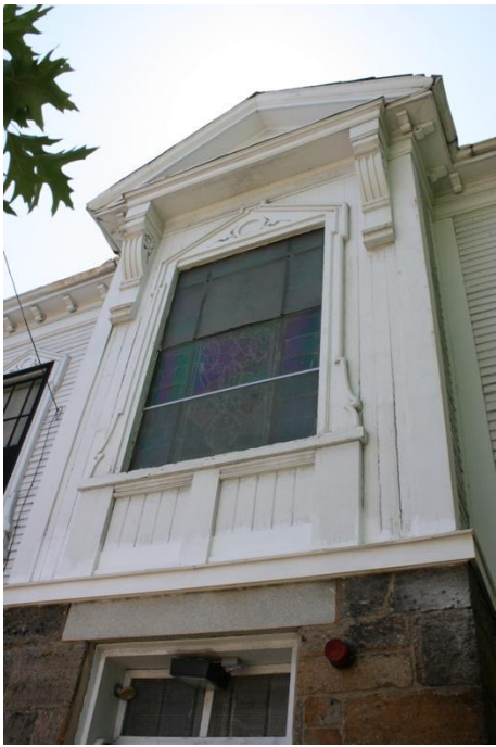
Figure 16. Putnam Chapel east elevation detail. June 2020.
