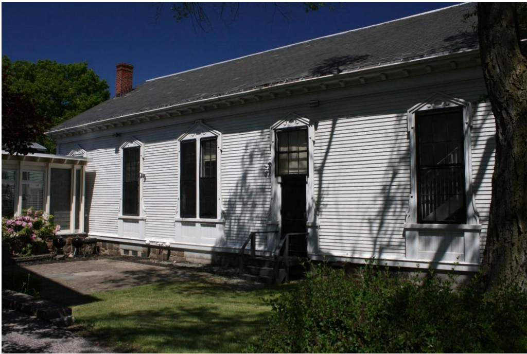
Figure 13. Putnam Chapel west elevation. June 2020.
