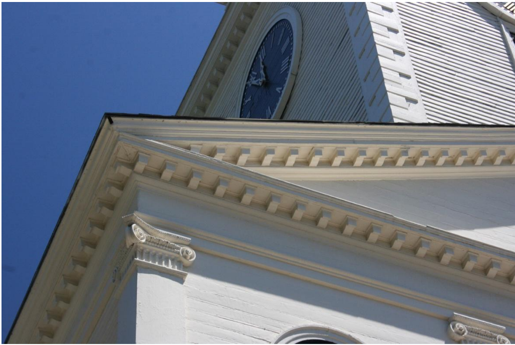
Figure 8. Meetinghouse eave detail at façade (west) elevation. June 2020.
