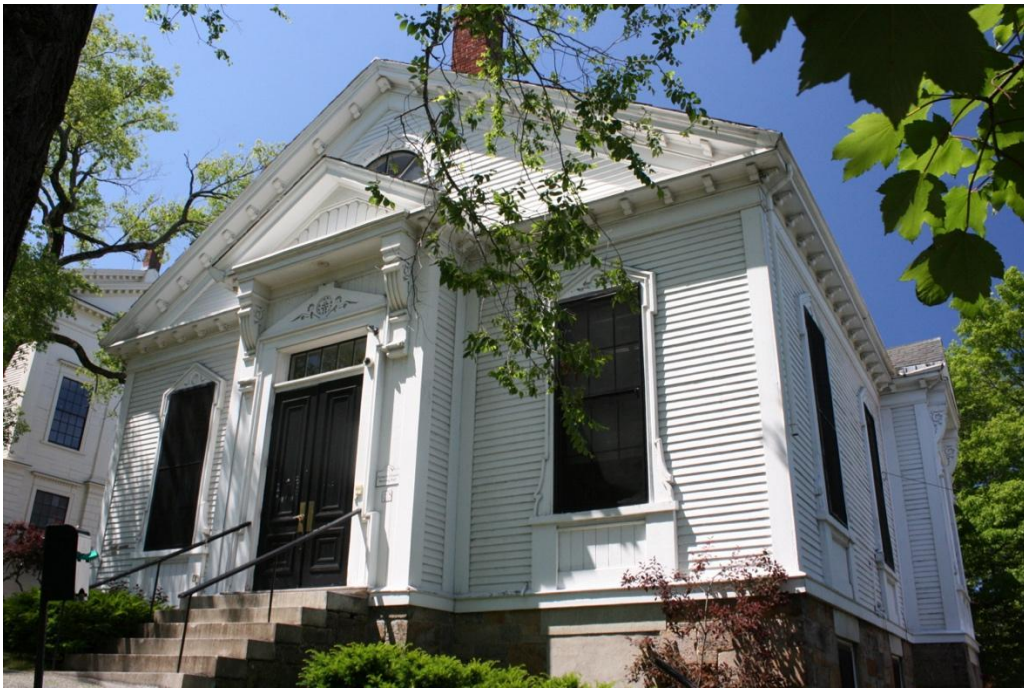
Figure 12. Putnam Chapel façade (south) and east elevations. June 2020.
