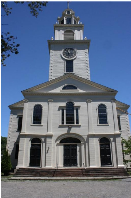
Figure 3. Meetinghouse façade (west) elevation. June 2020.
