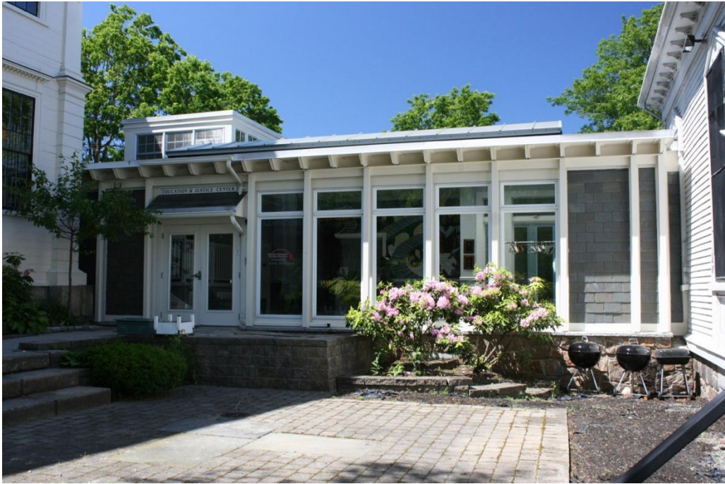
Figure 17. Education and Justice Center façade (south) elevation. June 2020.
