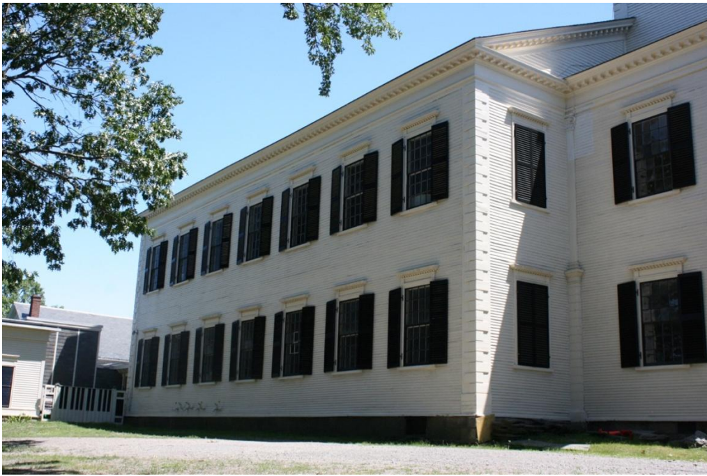
Figure 4. Meetinghouse north elevation. June 2020.
