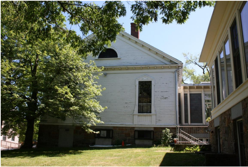
Figure 14. Putnam Chapel north elevation. June 2020.
