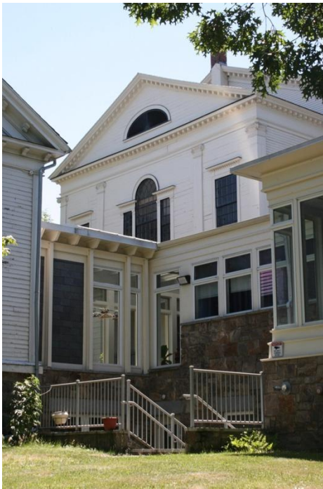
Figure 10. Interface of Chapel, Education and Justice Center, and Meetinghouse, looking southwest. June 2020.
