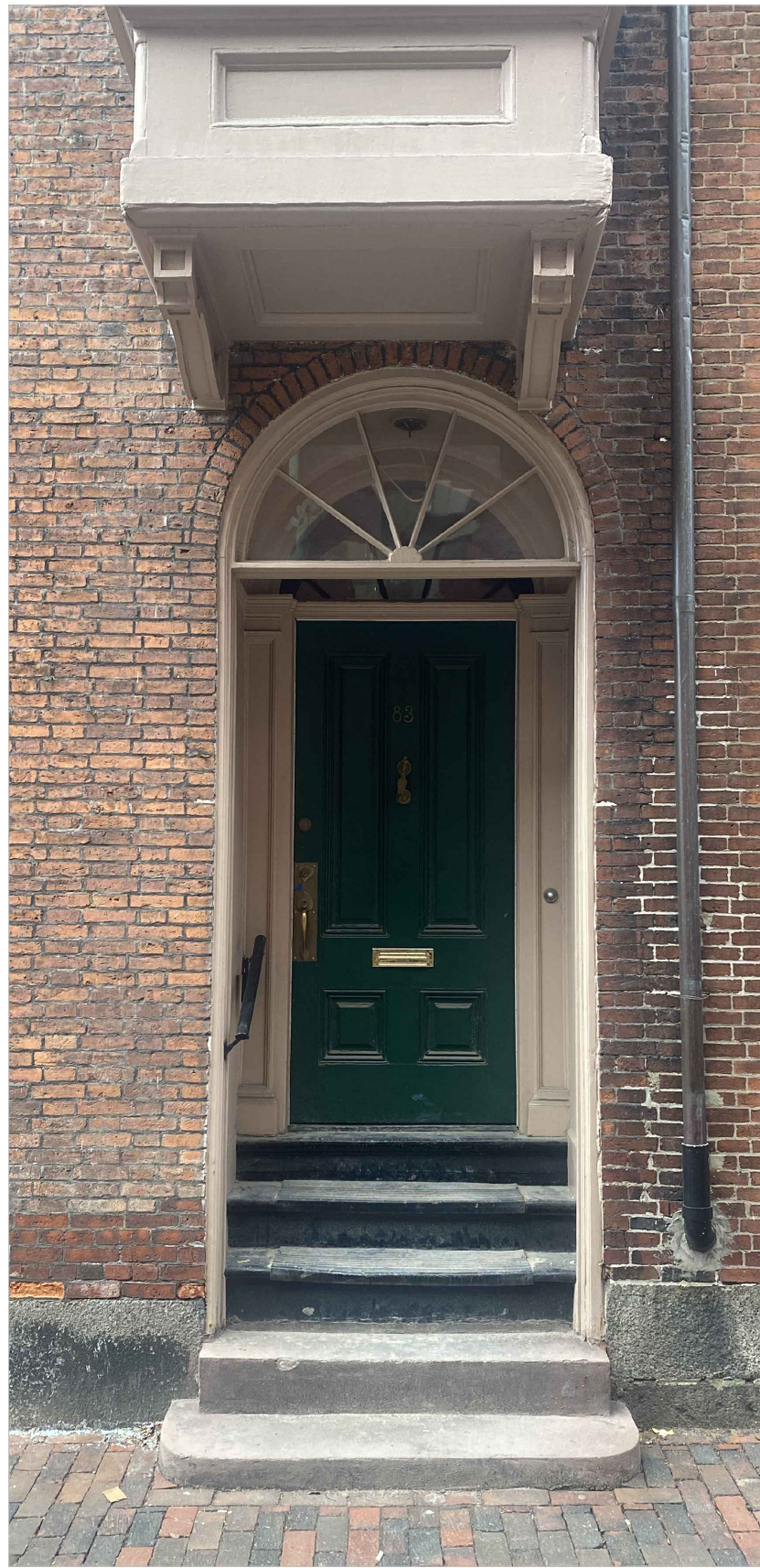
A EXISTING DOOR AND DOORBELL
