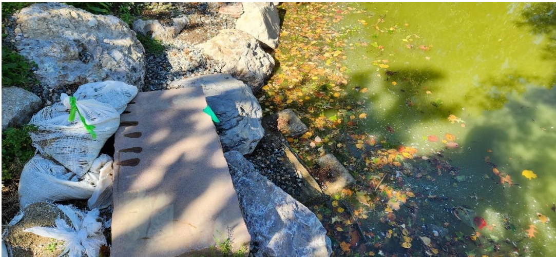
Outlet structure reinforcement. Photograph dated October 6, 2022.
