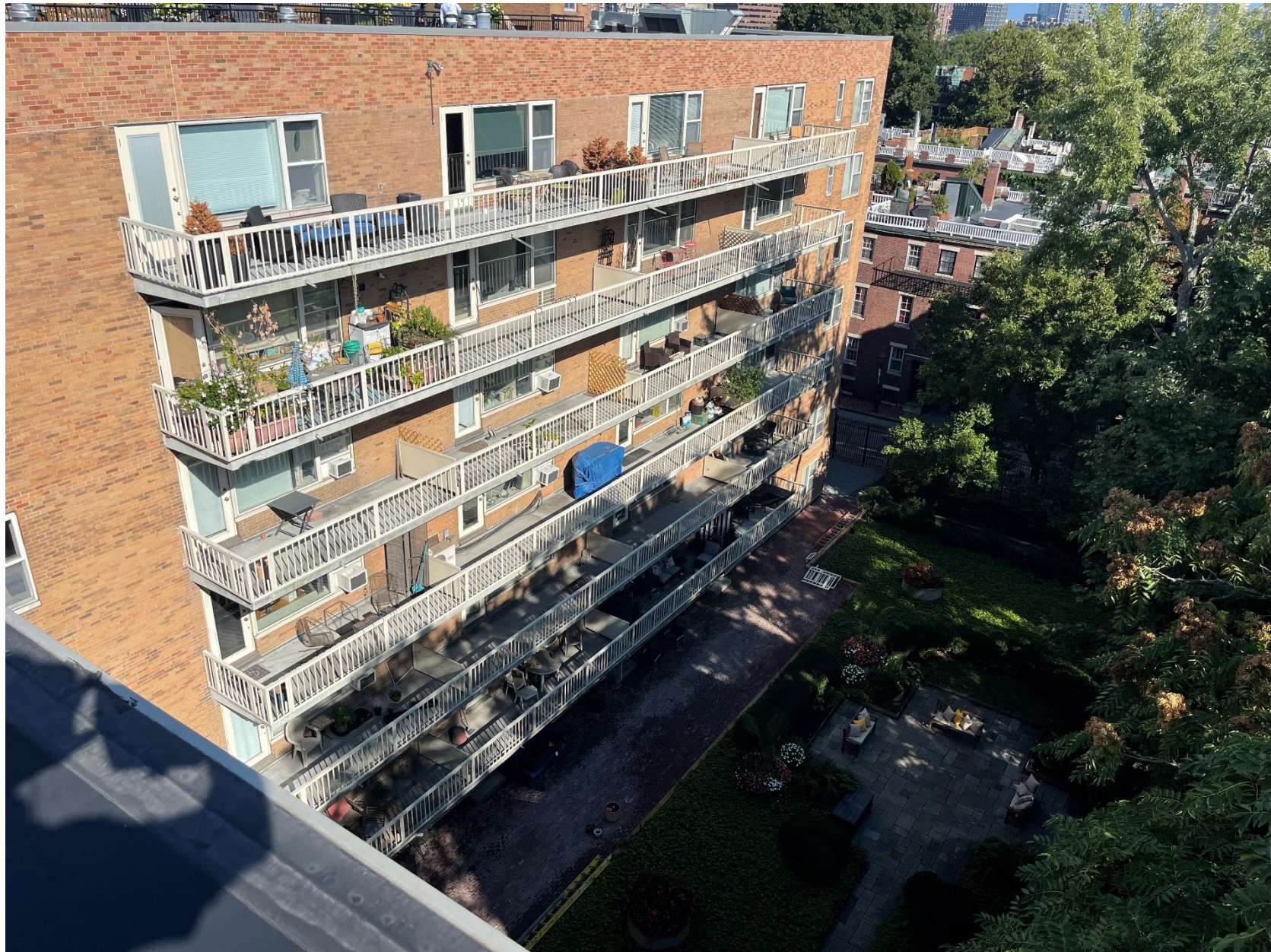
Existing/Typical Balcony Construction
