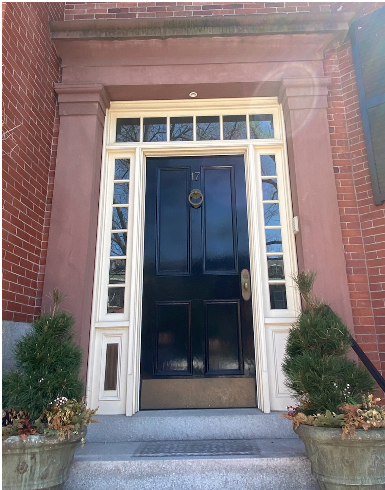
Front Entry Door - Repainting Only
