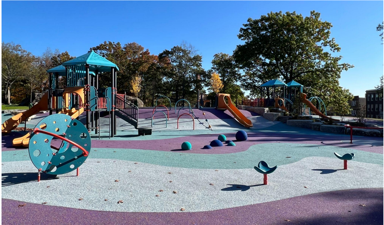
Playground equipment and surfacing installation
