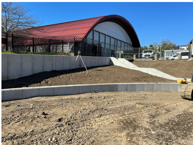
Field area walls
