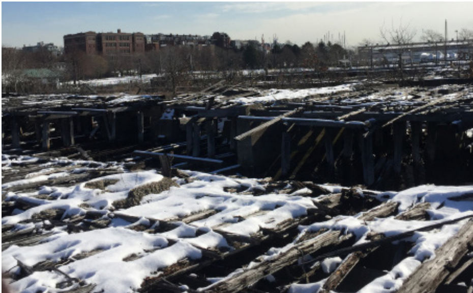
View 3: Looking Northeast across Project Site
