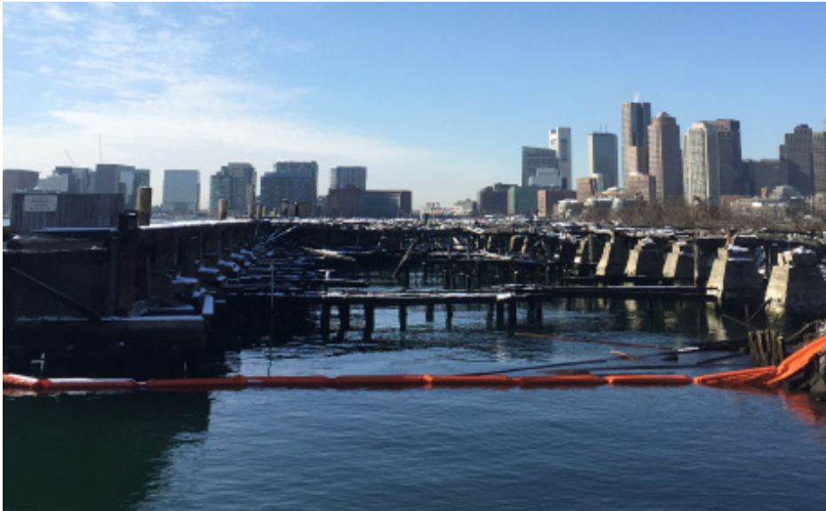
View 1: Looking Southwest toward Project Site
