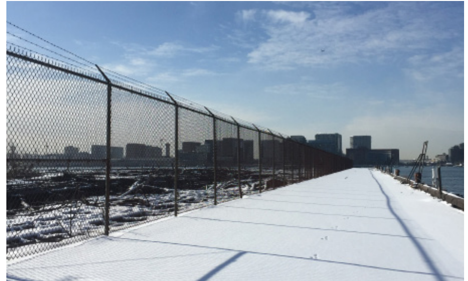
View 2: Looking Southwest along Concrete Apron
