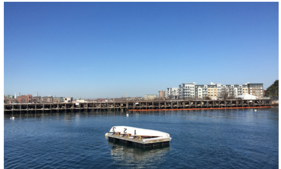
View 4: Looking Northwest toward Project Site
