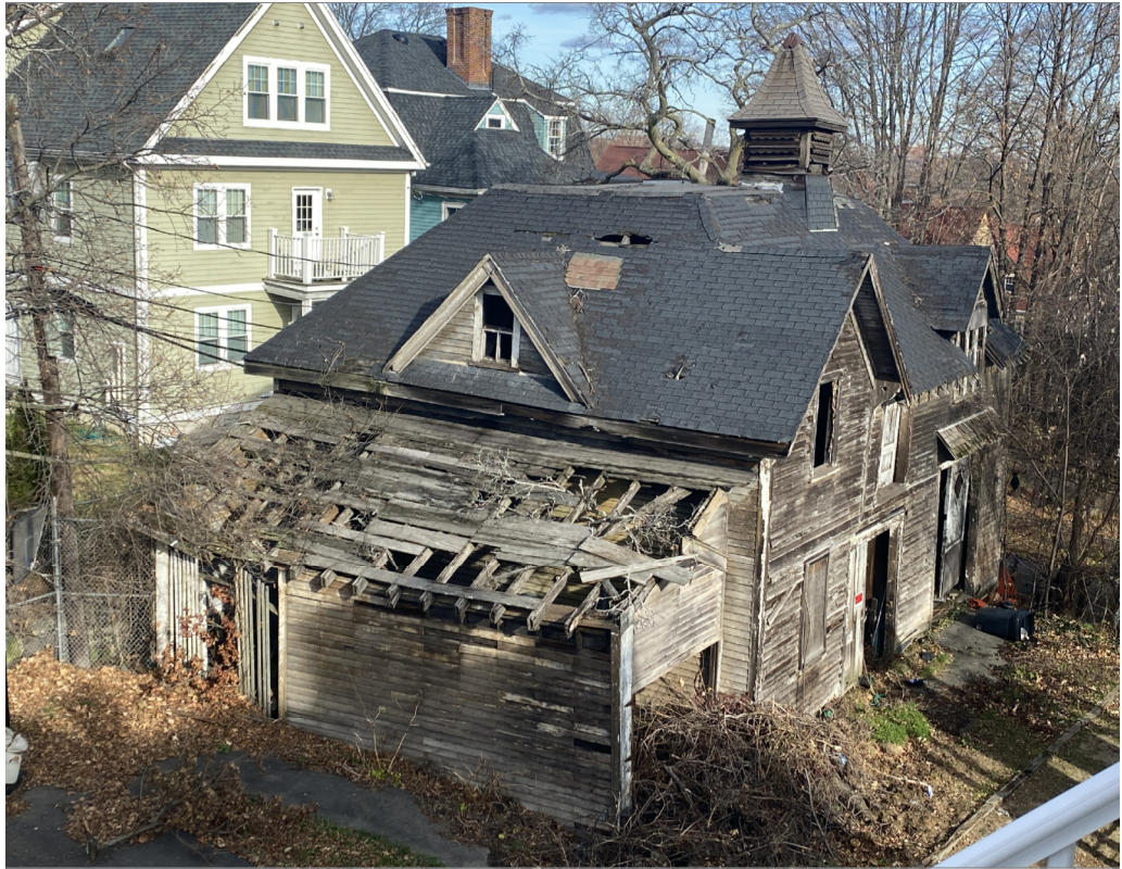
LEFT FACADE AND ROOF
