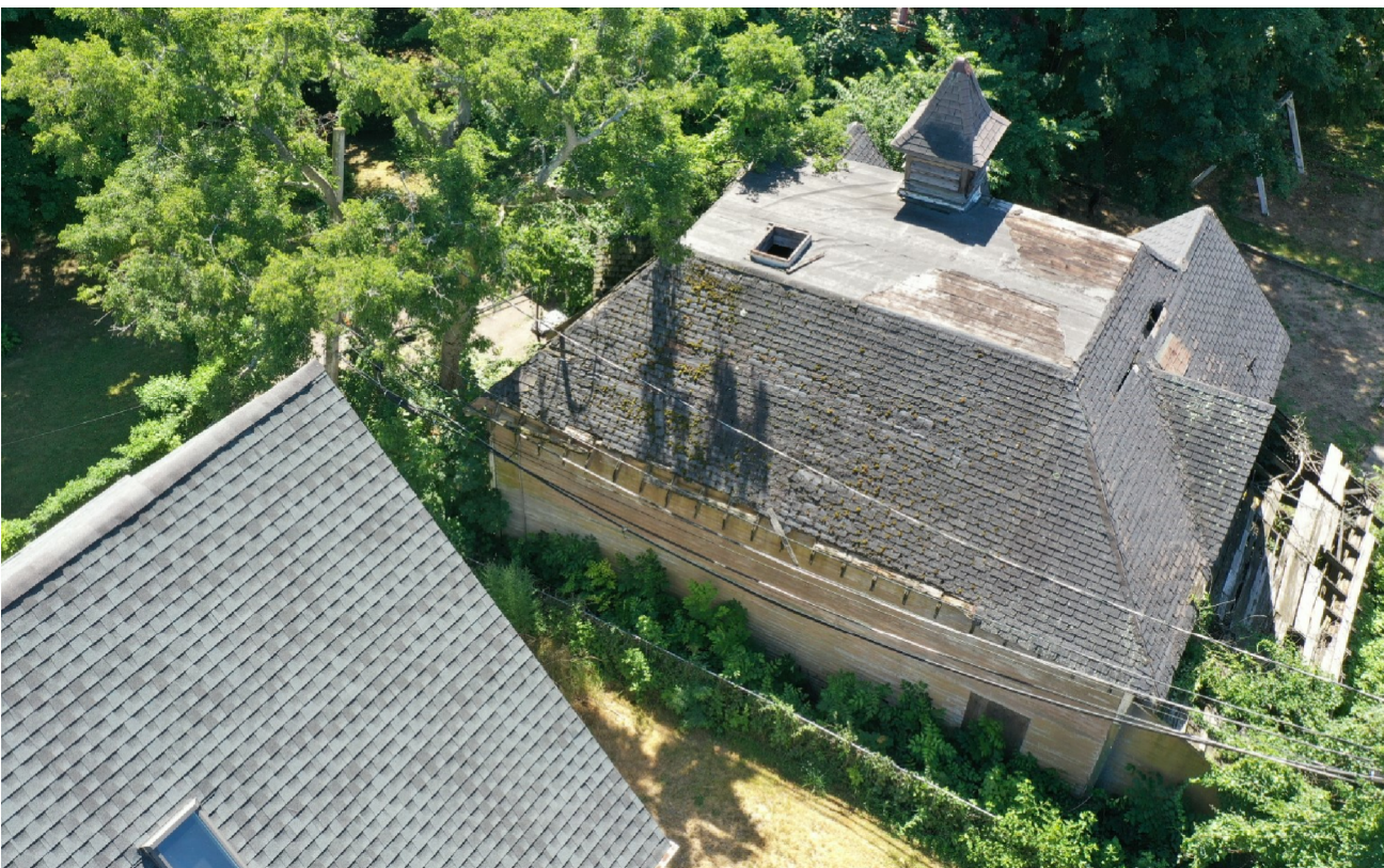
REAR FACADE AND ROOF
