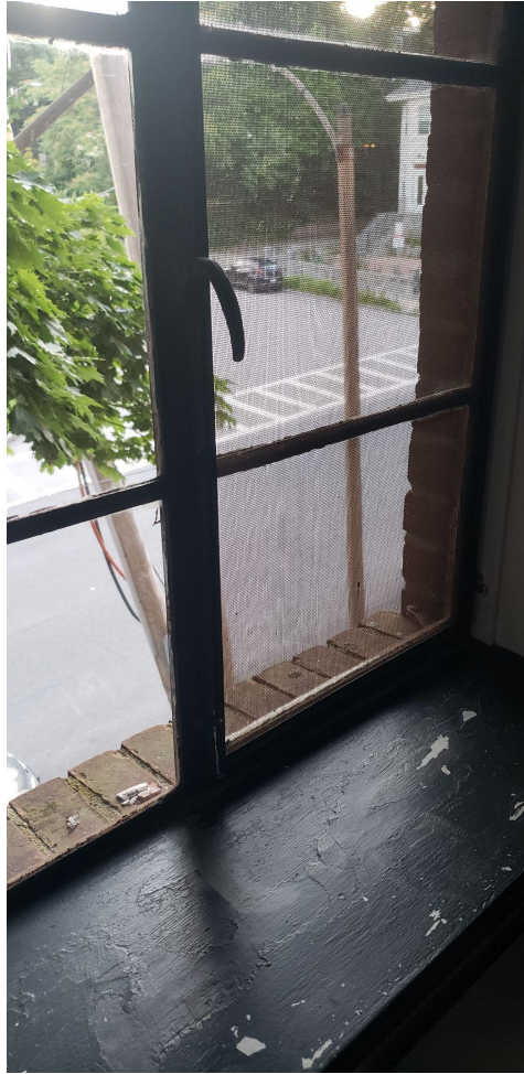
Interior window - some have gaps where bugs enter, some missing cranks to open, general wear & tear
