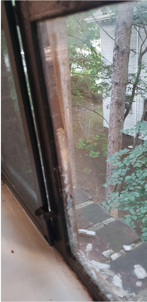
Interior window - some have gaps where bugs enter, some missing cranks to open, general wear & tear
