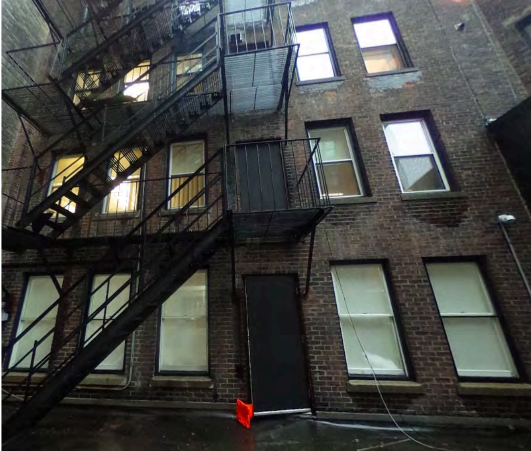
7 - 9 Newbury Street Rear Alley Roof Existing Fire Escape
