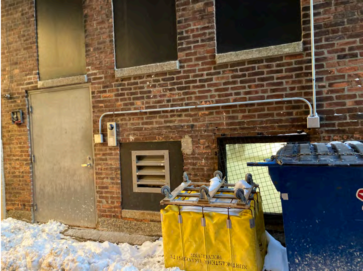
7 - 9 Newbury Street Rear Alley Existing Conditions
