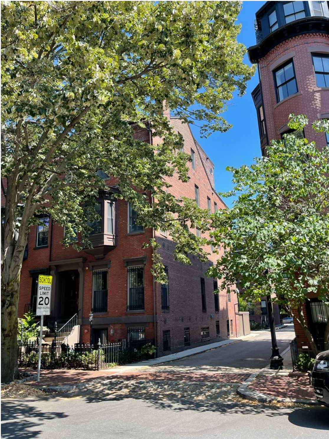
Right side view of 41 Worcester Street
