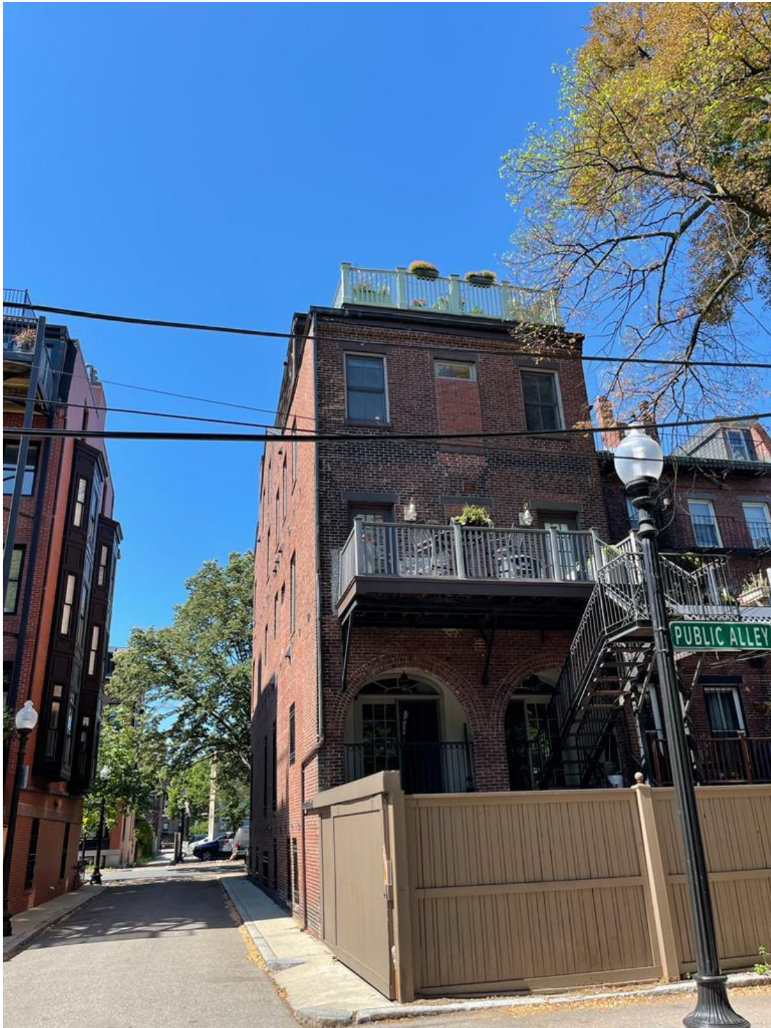
View of 41 Worcester St Roof deck from the public alley
