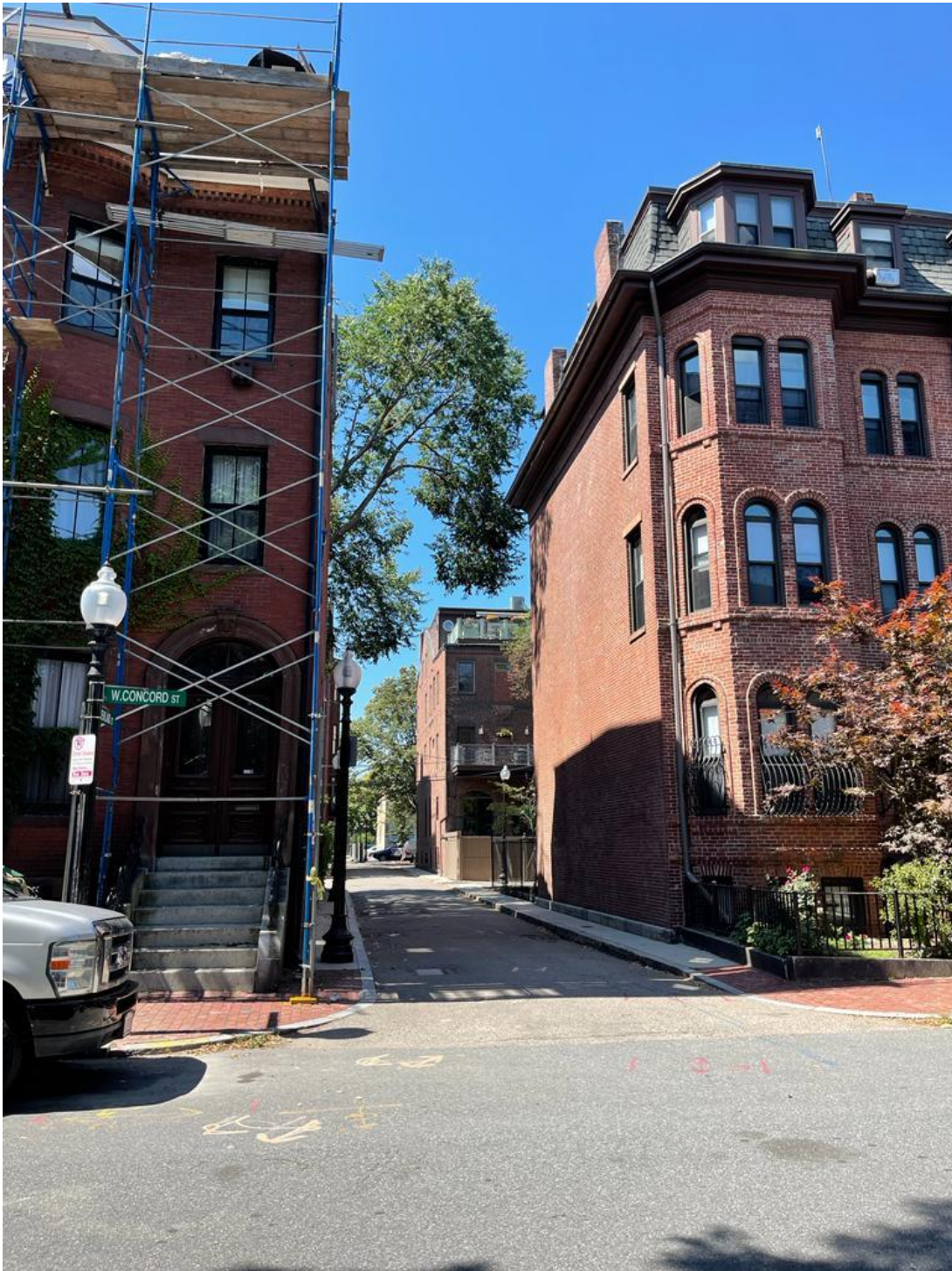
View of 41 Worcester St Roof deck from West Concord Street
