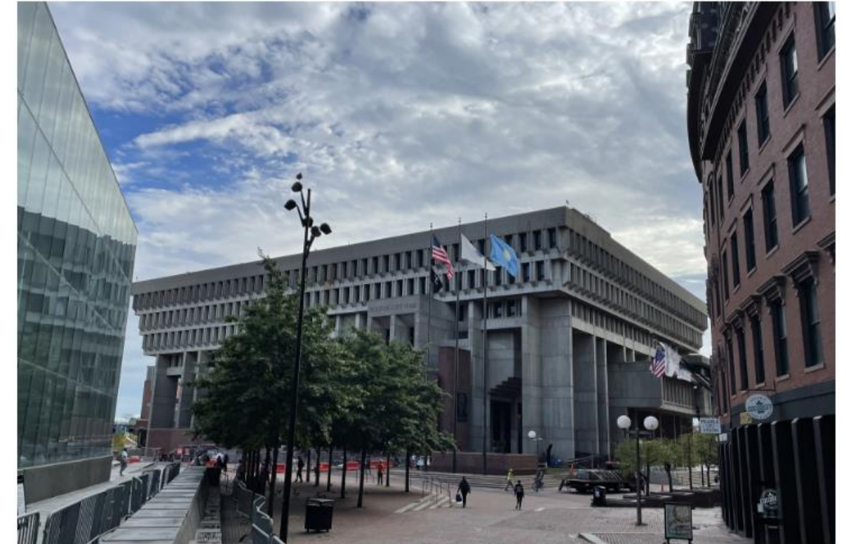
EXISTING PERSPECTIVE SHOWING CURRENT CONDITIONS
