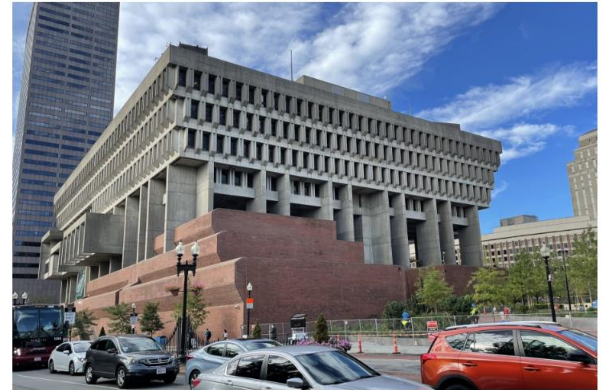
EXISTING PERSPECTIVE SHOWING CURRENT CONDITIONS
