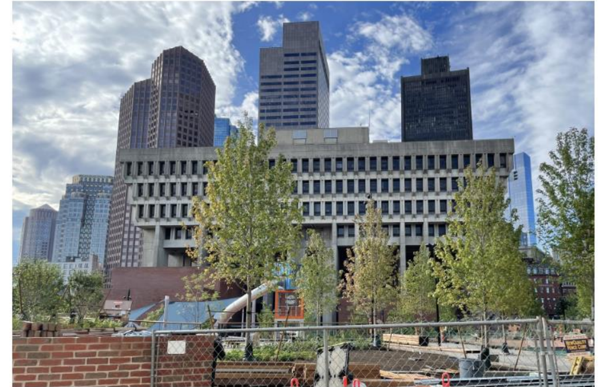
EXISTING PERSPECTIVE SHOWING CURRENT CONDITIONS
