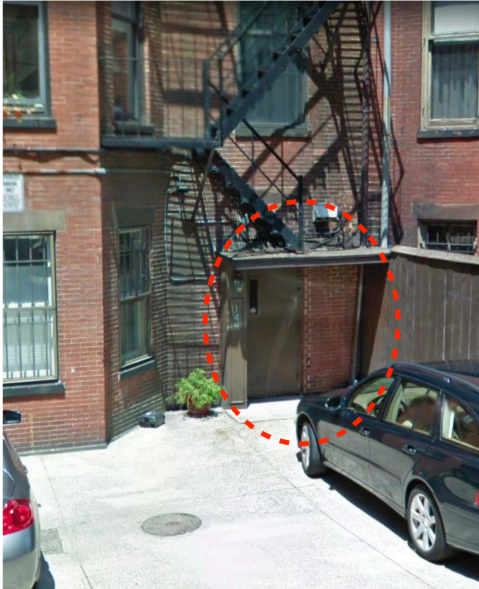
EXISTING REAR DOORWAY @ PROPOSED LOCATION
