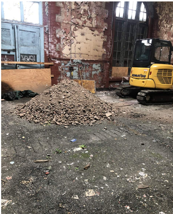
Photograph No. 9: Excavated material from test pit.
