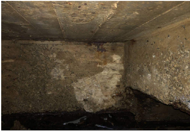
Photograph No. 5: View beneath cast-in-place slab of void.
