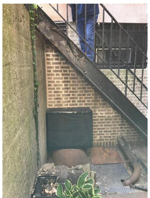
4.) Pic below is of mock up of A/C condenser shown in proposed installation location below exterior stairs at back of 68 Beacon St. Unit stock color is "Sandstone."
