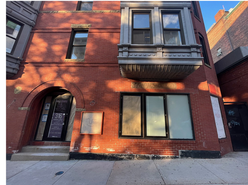
EXISTING CONDITIONS IMAGE
