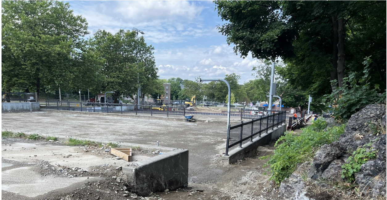
Basketball Court preparation
