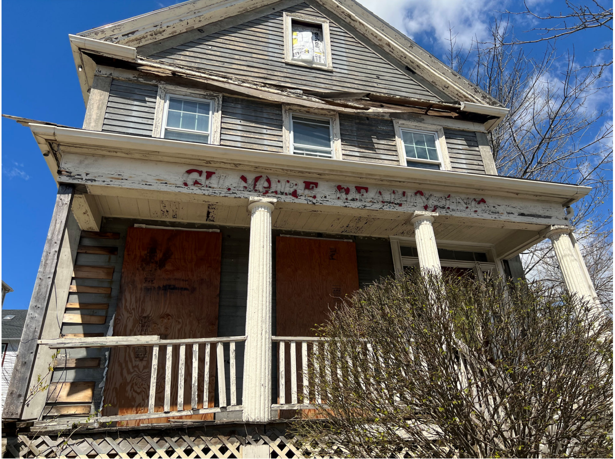
Figure 4. Façade close-up, April 22, 2022.
