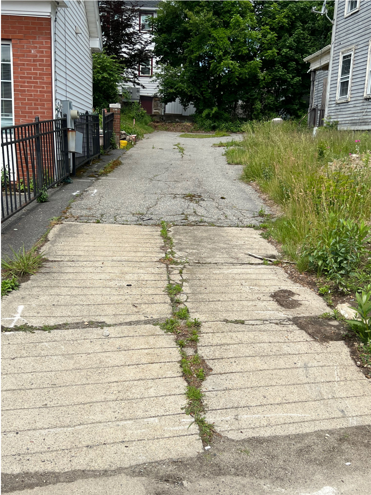
Figure 8. South elevation showing concrete and asphalt driveway, April 22, 2022
