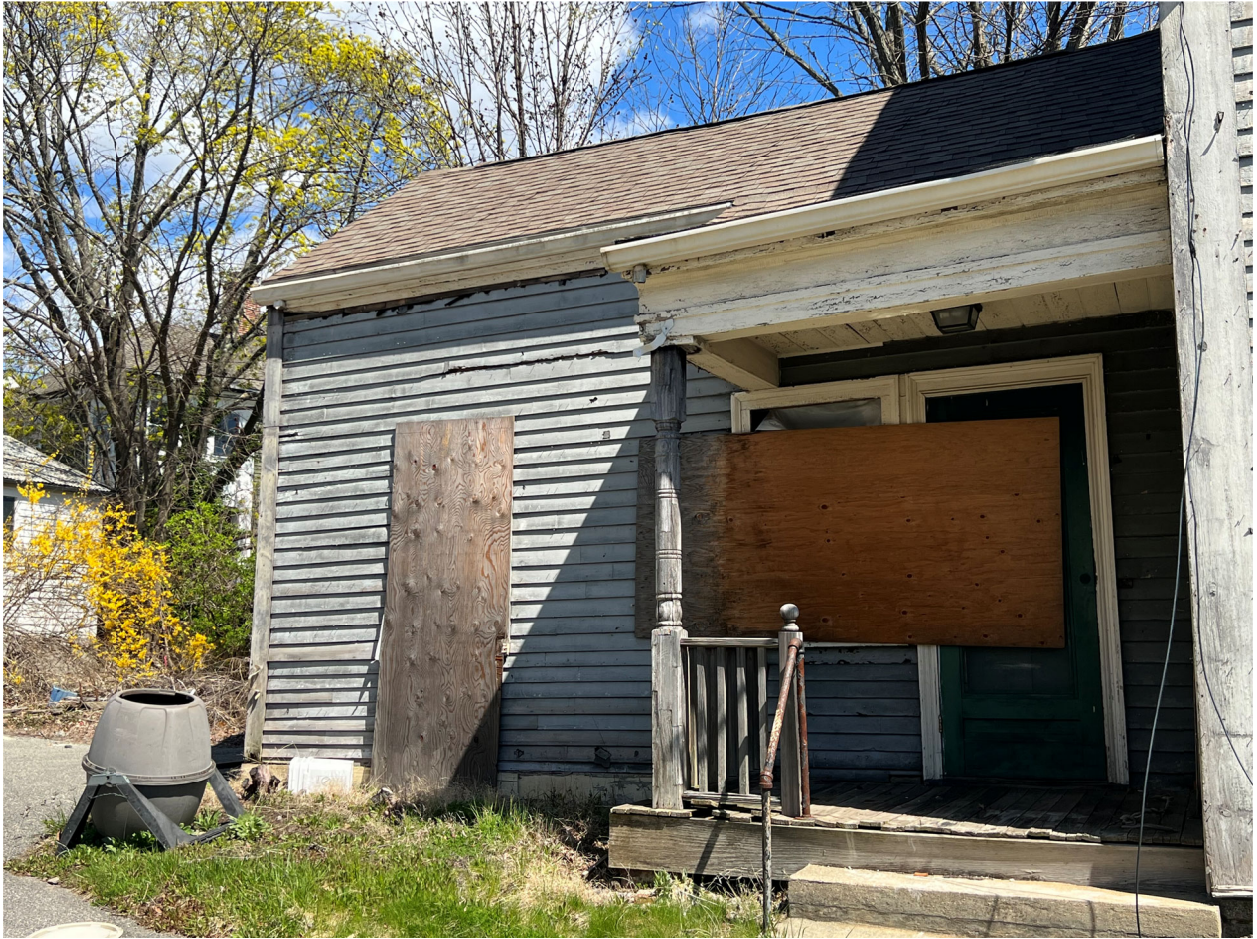
Figure 10. Back porch and side of ell, south elevation, April 22, 2022.
