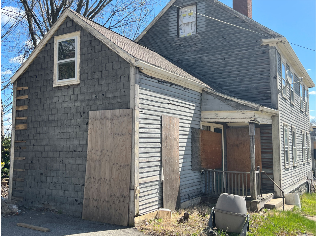
Figure 11. West elevation (rear) showing ell and back porch, April 22, 2022.
