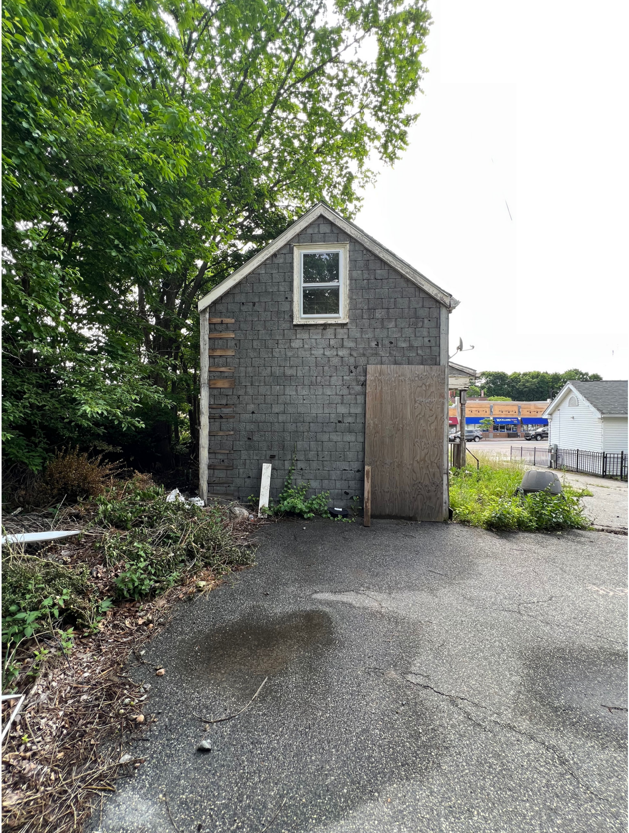
Figure 12. West elevation, asbestos-shingled ell with boarded entrance.
