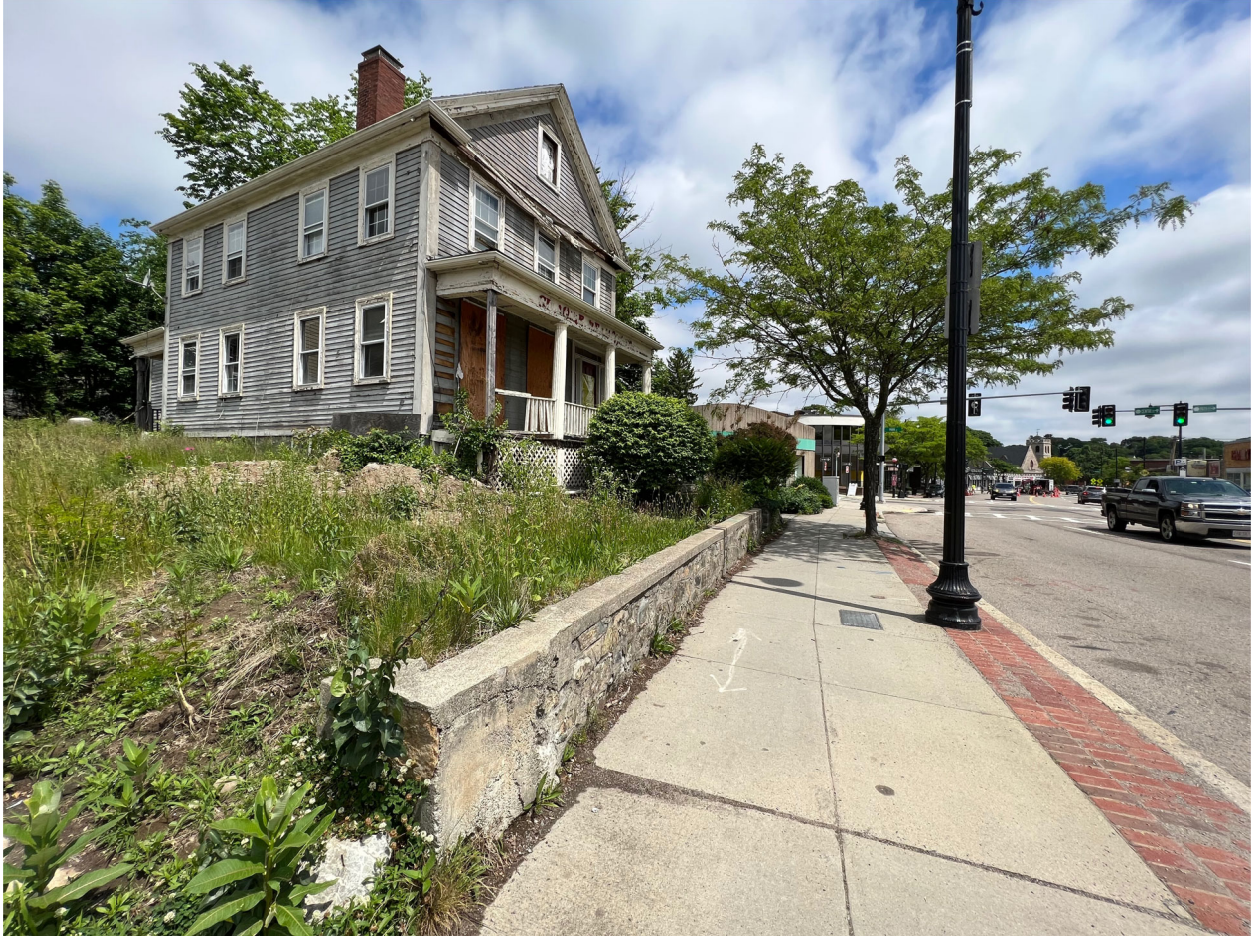
Figure 3. Frontage retaining wall, taken from the southerly end of the property looking north on Centre Street, June 2, 2022.
