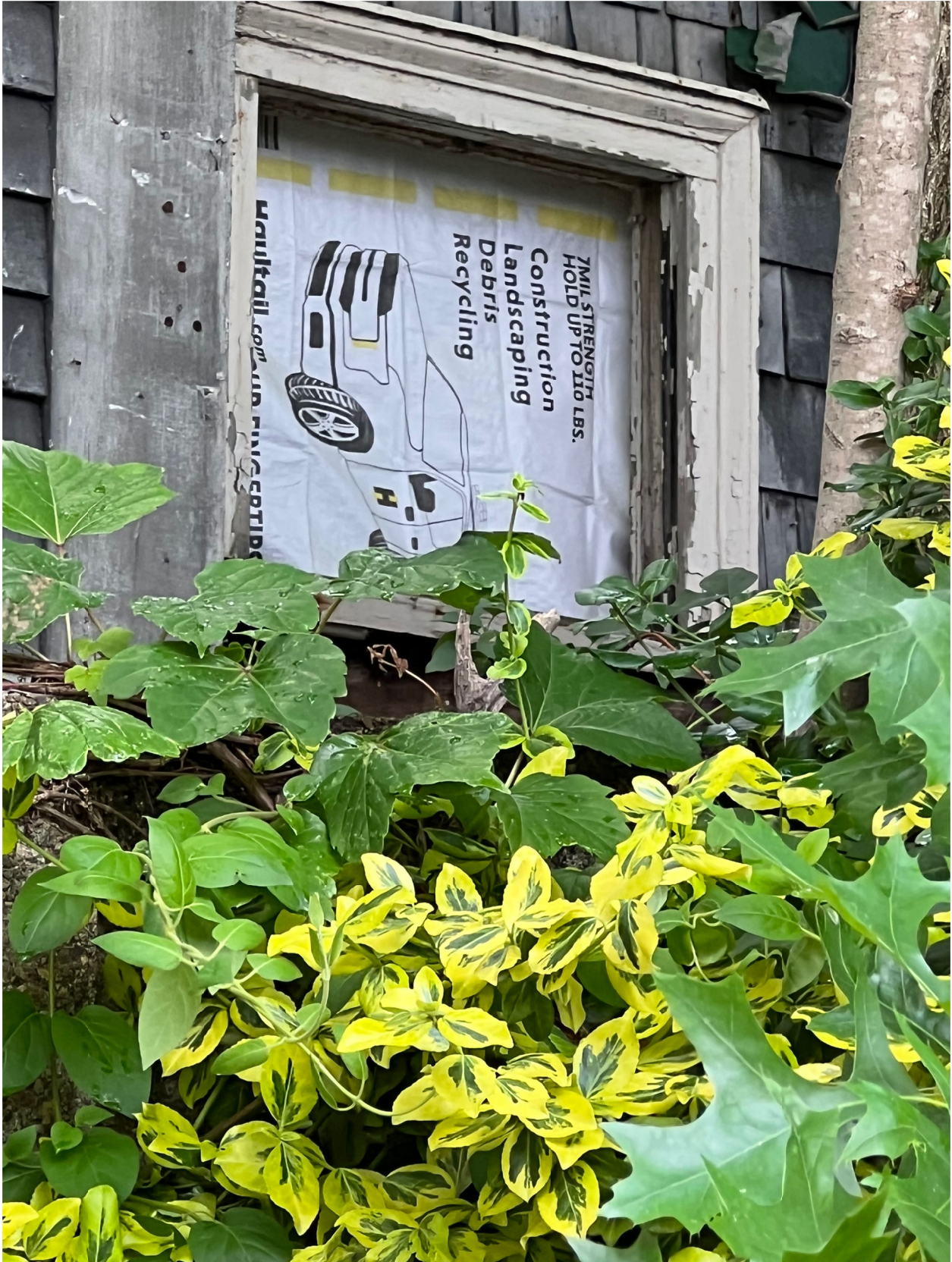
Figure 16. Closeup of ell window, north elevation, taken June 2, 2022.
