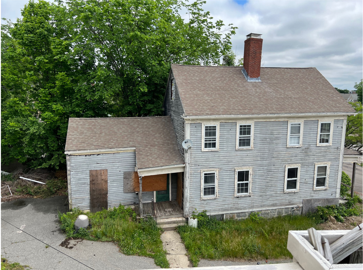
Figure 17. South elevation showing roof, taken from second-floor deck of abutting property at 3 Richwood Street, June 2, 2022.
