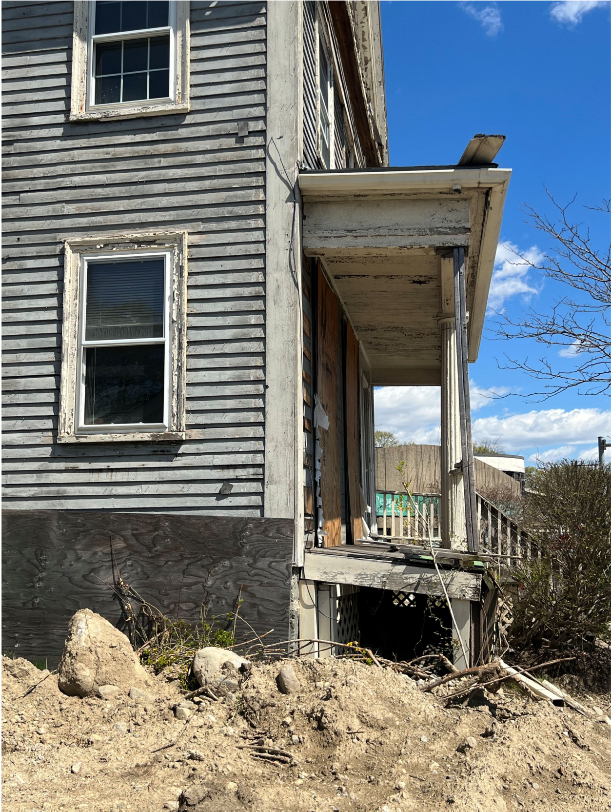
Figure 6. Side view of façade porch, taken at south elevation, April 22, 2022.
