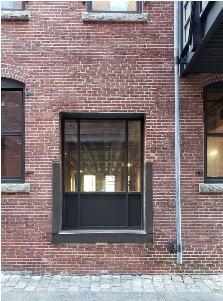
VIEW OF EXISTING OPENING
