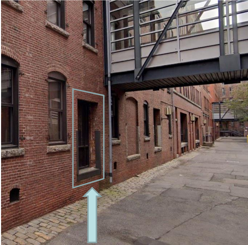
REAR OF BUILDING - ALLEY VIEW
