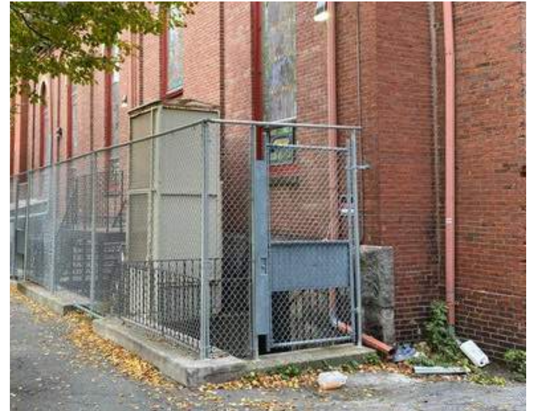
EXTERIOR LIFT TO LEVEL 1
