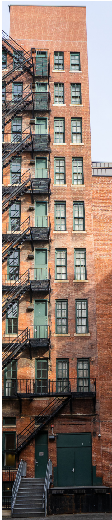
EXISTING ELEVATOR SHAFTWALL AT 51 MELCHER
