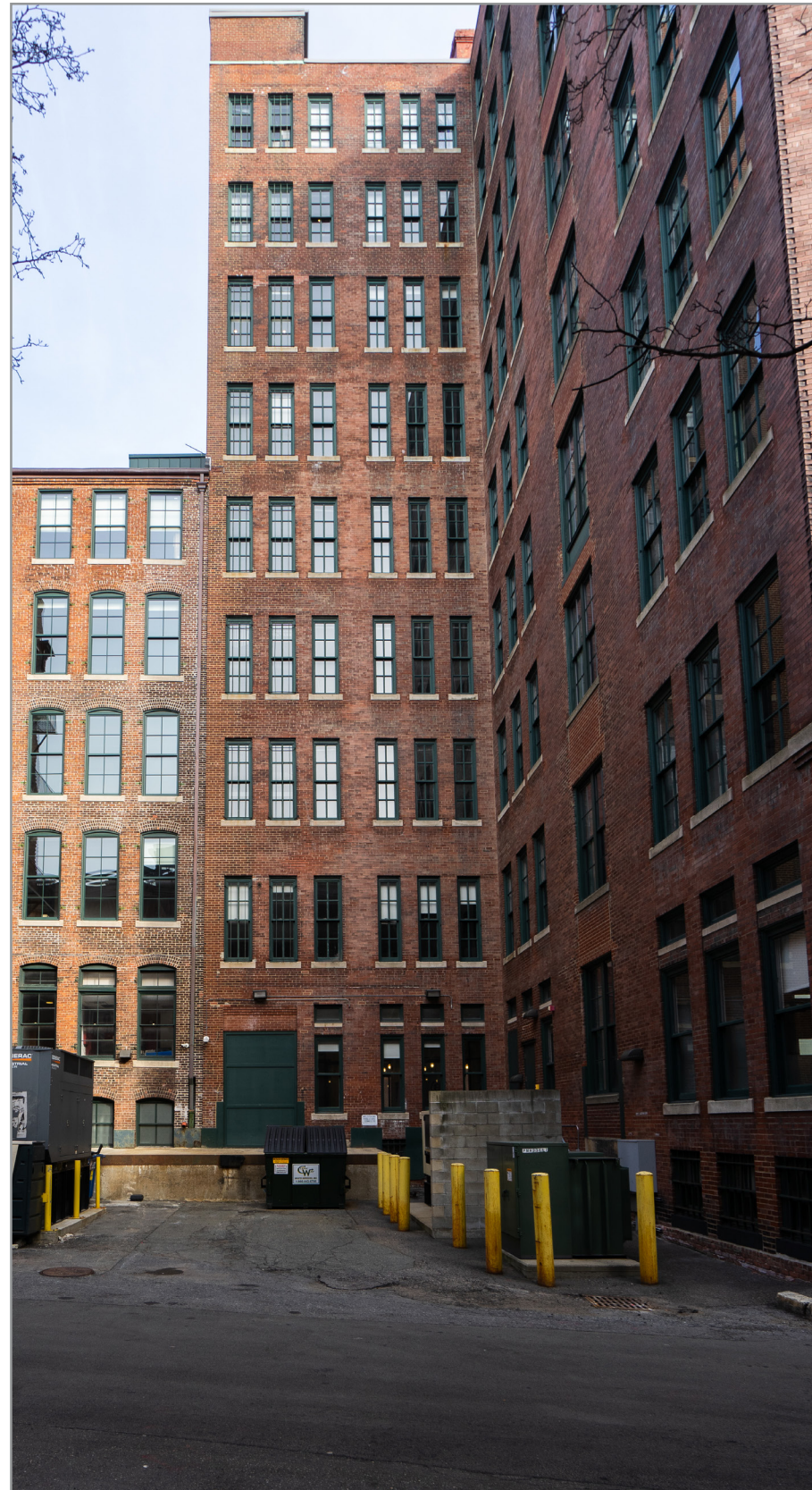
EXISTING PHOTOGRAPH - LOADING BAY
