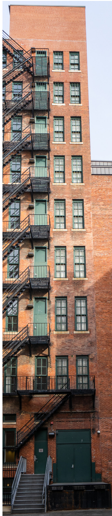
EXISTING ELEVATOR SHAFTWALL AT 51 MELCHER
