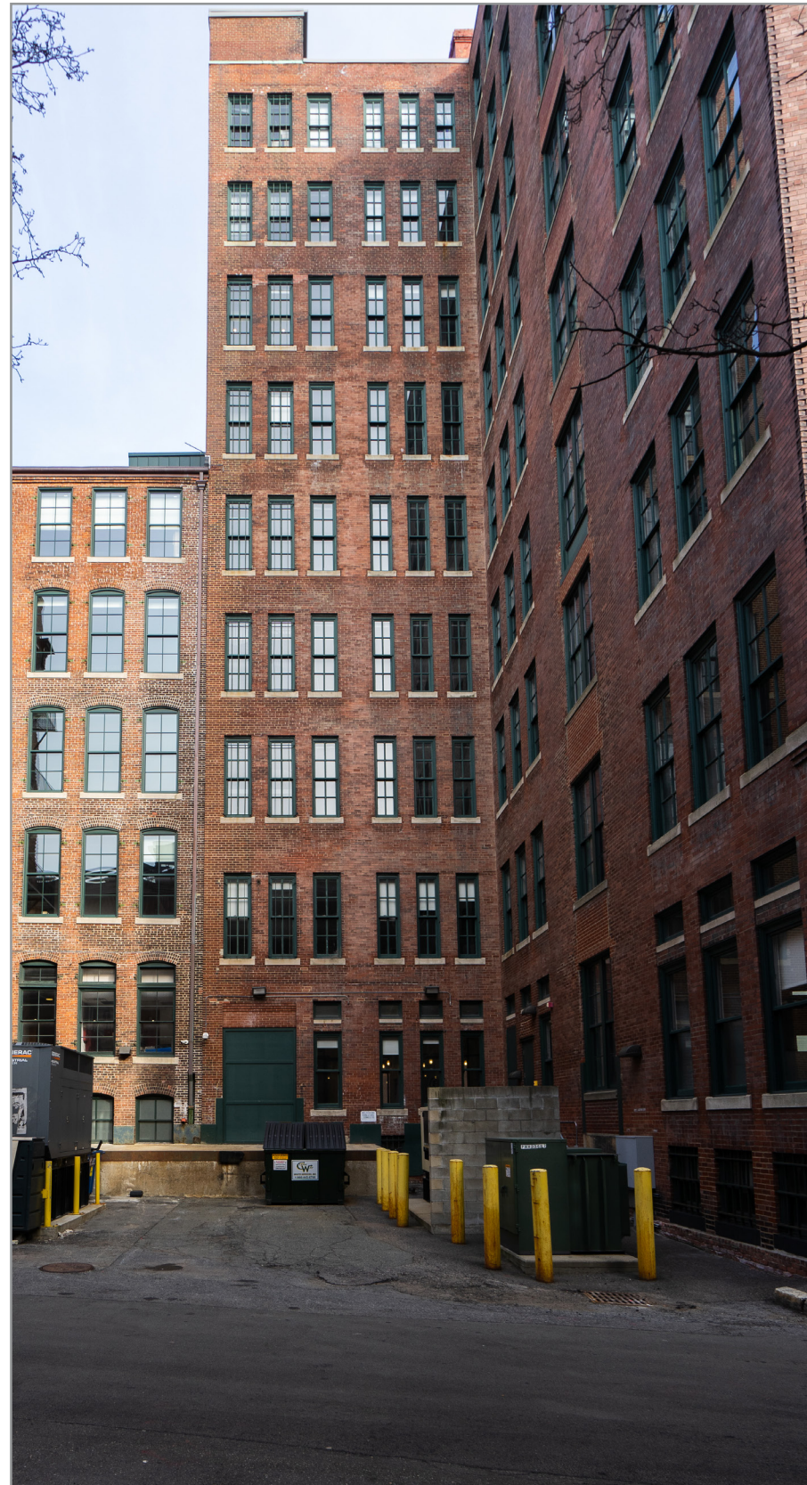
EXISTING PHOTOGRAPH - LOADING BAY
