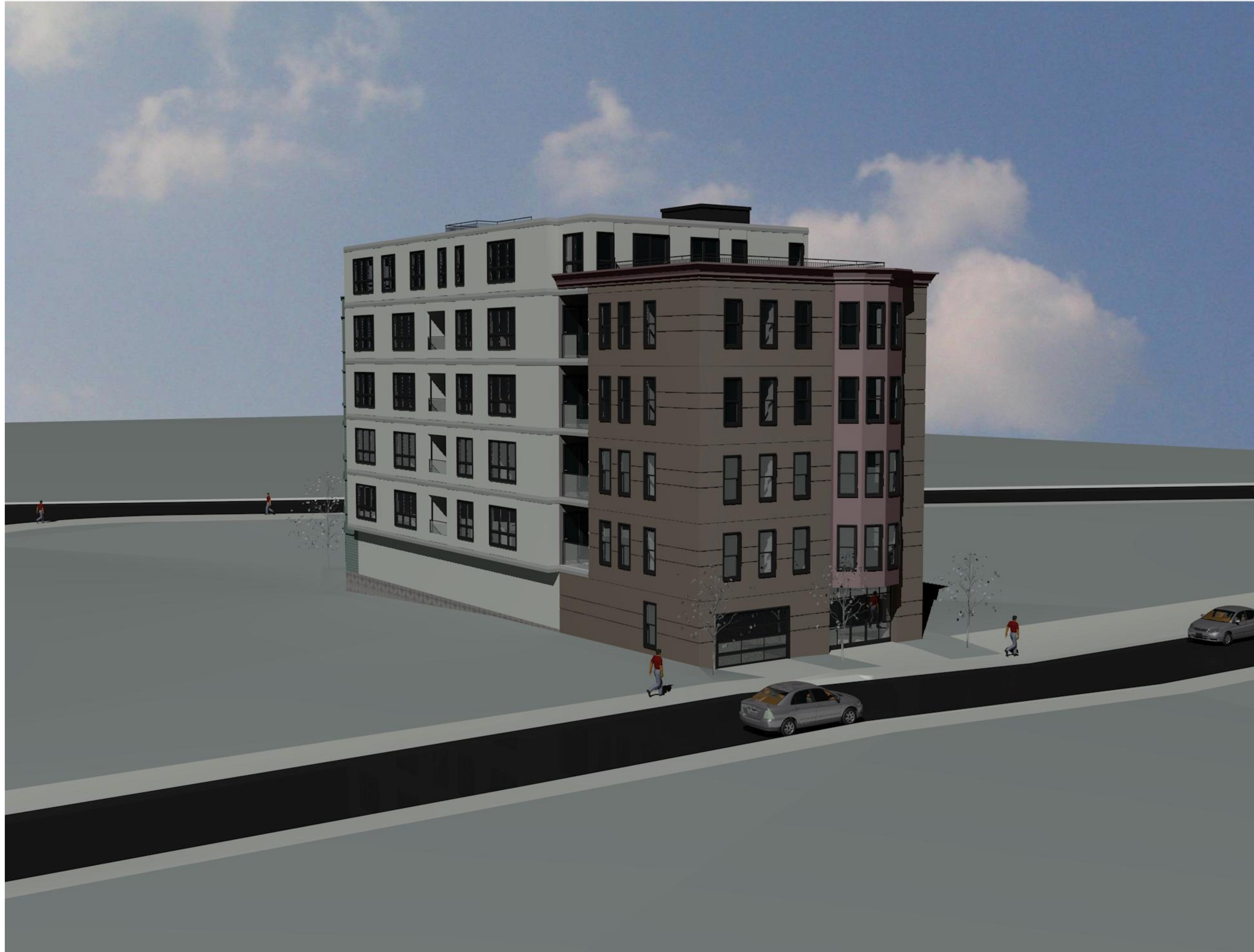
STREET VIEW LOOKING SOUTHEAST
